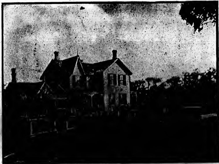
"THE WILLOWS" — SIDE VIEW, RESIDENCE OF W. C. COMMINS.
