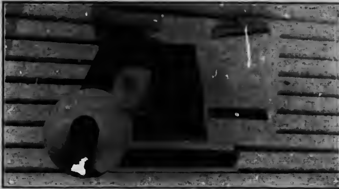
Fig. 9. Cold-air intake and hood for "Iceless Refrigeration." The adjacent door is used in ventilating the packing-house when it is also used as a storage.
