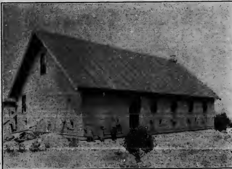
Fig. 5. A Wenatchee Valley fruit storage built by Dr. Whitney, of Cashmere, Wash. Note the ventilating system.
