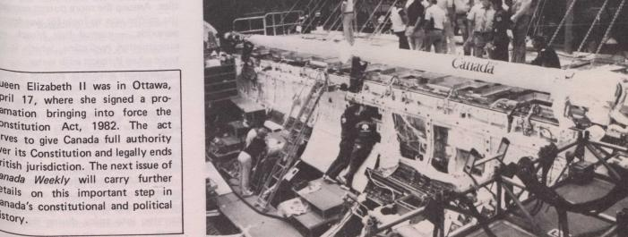
Canadarm, wrapped in its white thermal blanket, is placed on shuttle orbiter Columbia prior to shuttle's second mission.
