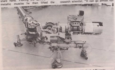
View of Canadarm, with wrist joint in the forefront, at Spar Limited of Toronto.
