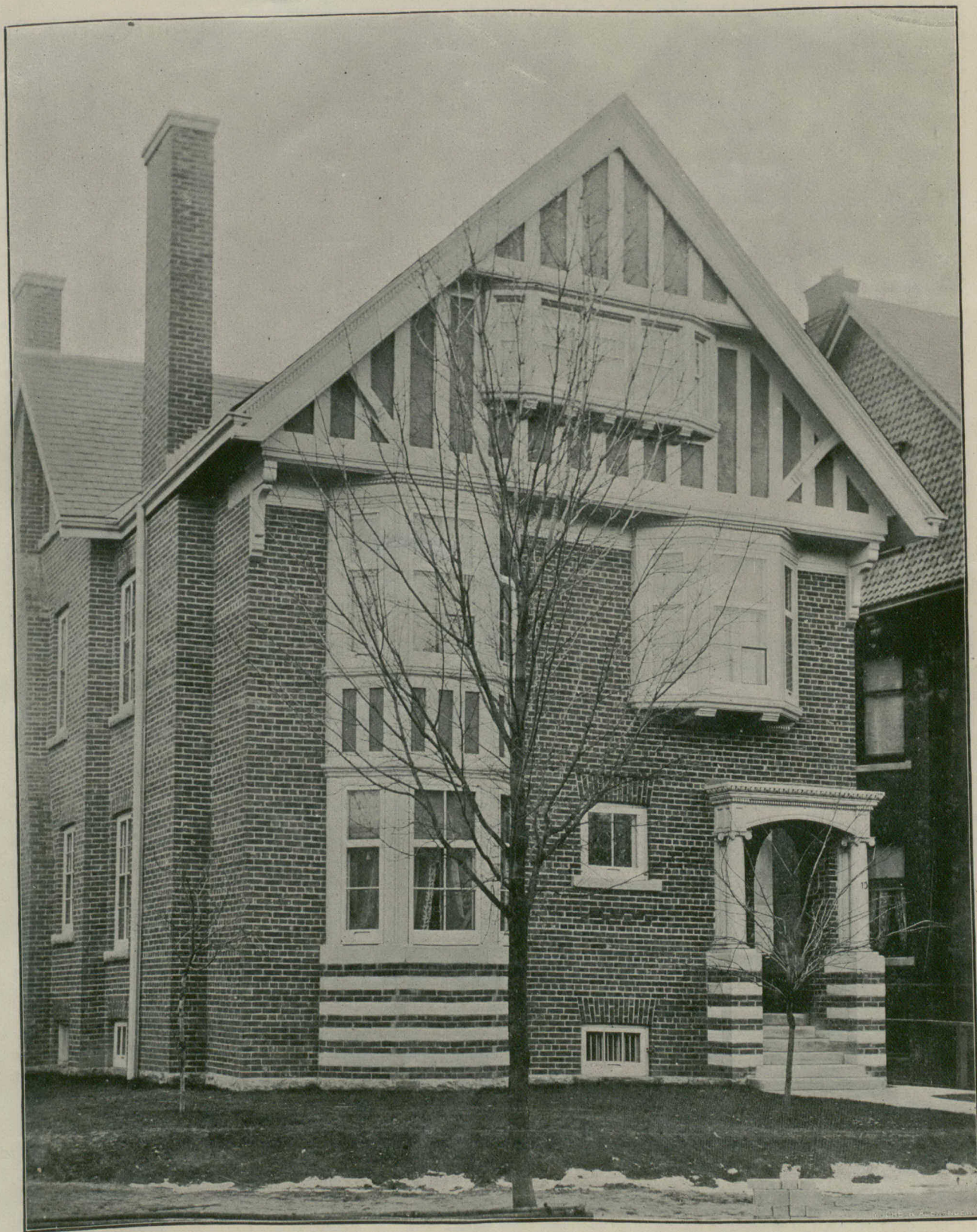
RESIDENCE OF MR. W. P. GUNDY, 13 MAPLE AVENUE, TORONTO. MR. F. S. BAKER, F.R.I.B.A., ARCHITECT.
