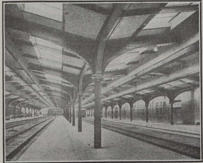
Interior View of Ottawa Train Shed.
