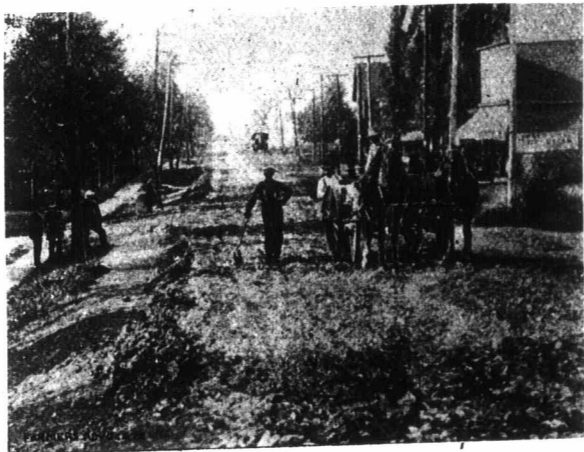
FIG. II.—ROADBED WITH FIRST LAYER OF BROKEN STONE, BEFORE BEING ROLLED.
