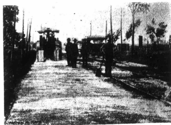
FIG. III.—PORTION OF ROAD ALMOST FINISHED.
