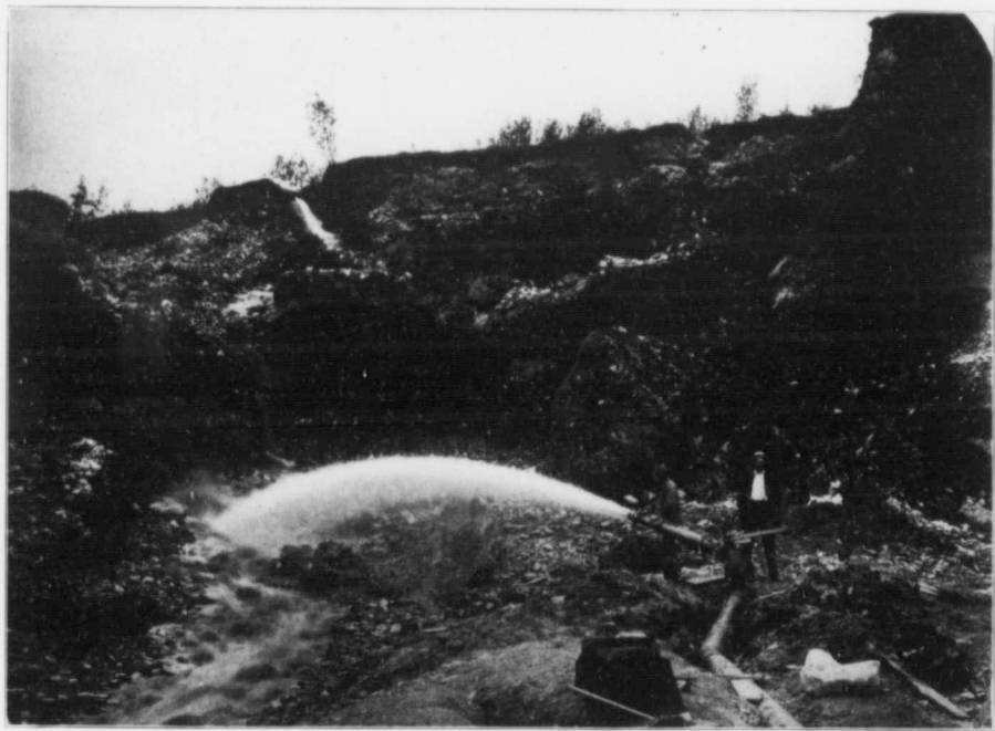
HYDRAULIC WORK ON FRENCH HILL, Y. T., 1908.
