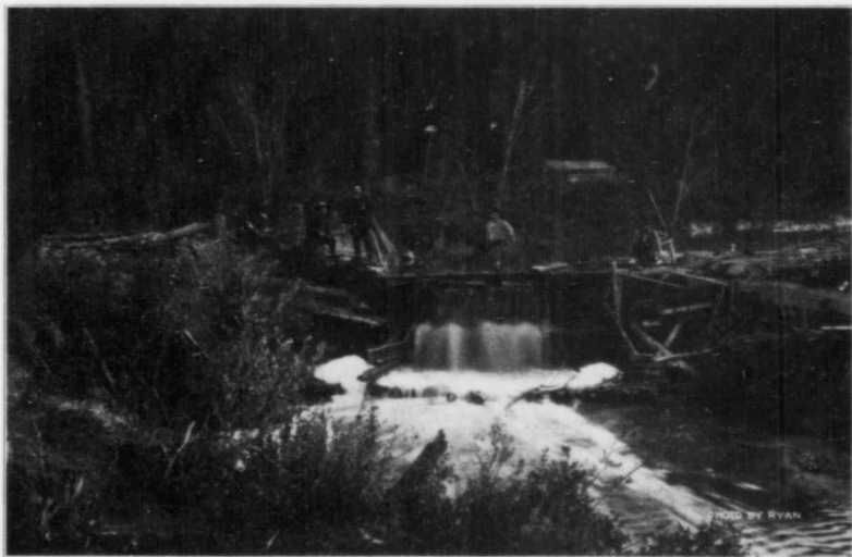
WATER DAM ON 69 BELOW HUNKER CREEK, Y. T.
