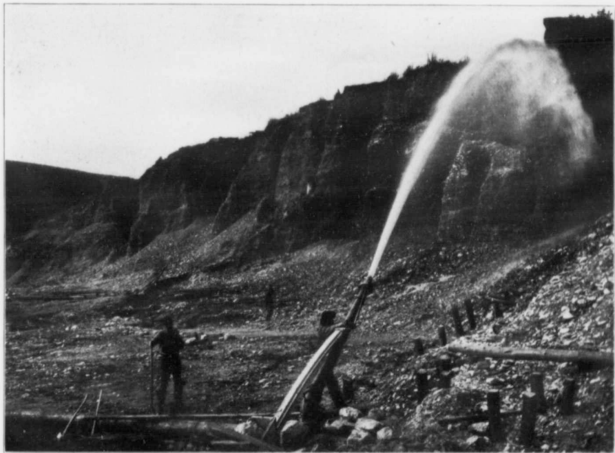
HYDRAULIC WORK ON FRENCH HILL, Y. T.
