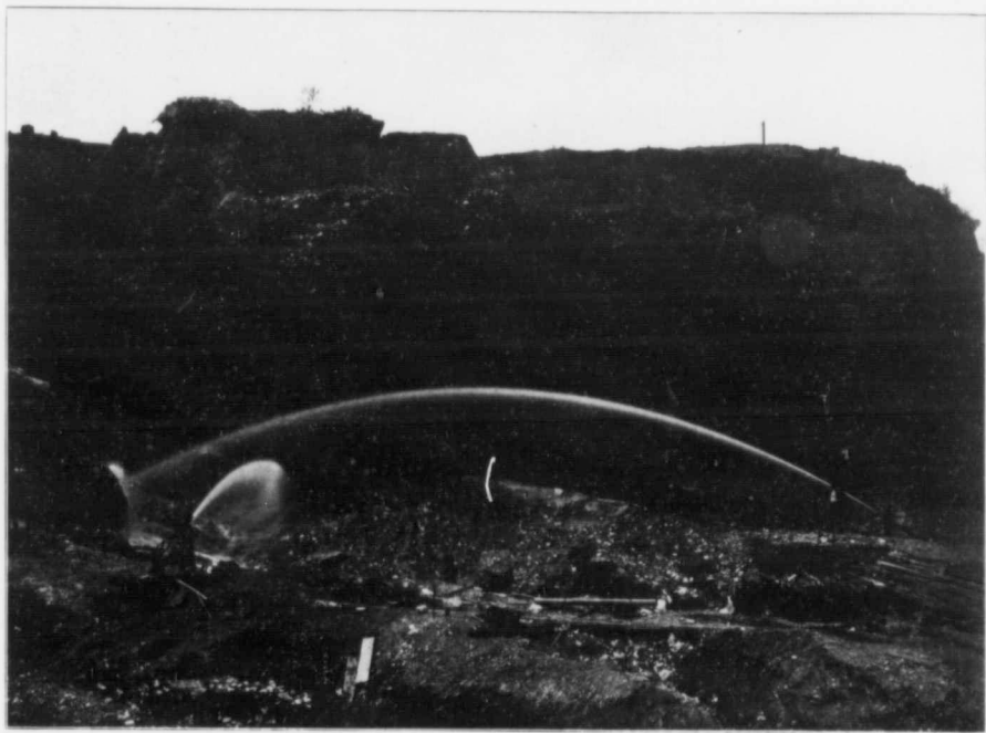
HYDRAULIC WORK ON FRENCH HILL, Y. T., 1908.
