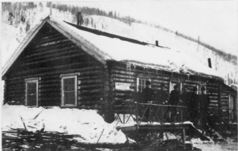
N. W. M. POLICE STATION, GOLD BOTTOM, Y. T.
