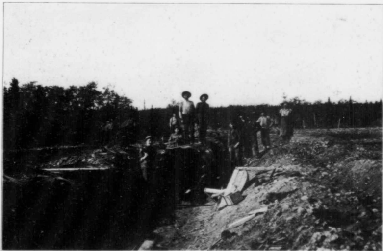
CONSTRUCTION 12 MILE PIPE LINE, Y. T.
