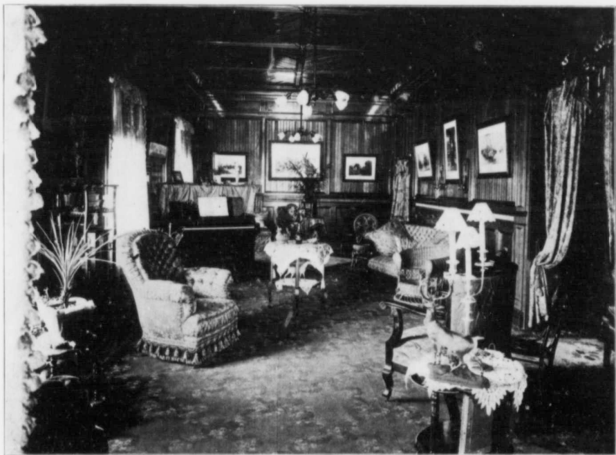
INTERIOR VIEW, COMMISSIONER'S RESIDENCE, DAWSON, Y. T.
