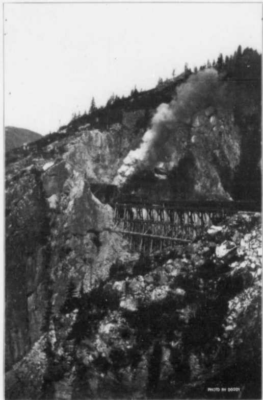
16 MILES FROM SKAGWAY, W. P. RAILROAD.
