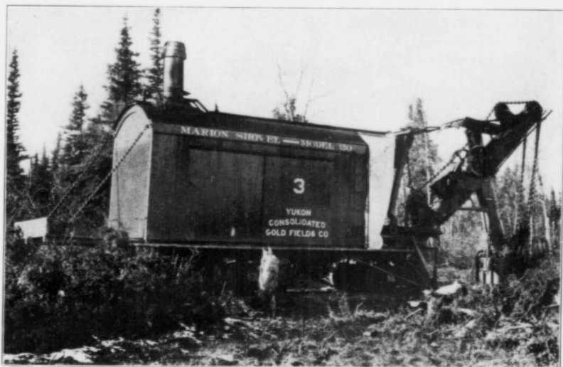
STEAM SHOVEL ON THE TWELVE MILE DITCH, YUKON TERRITORY.
