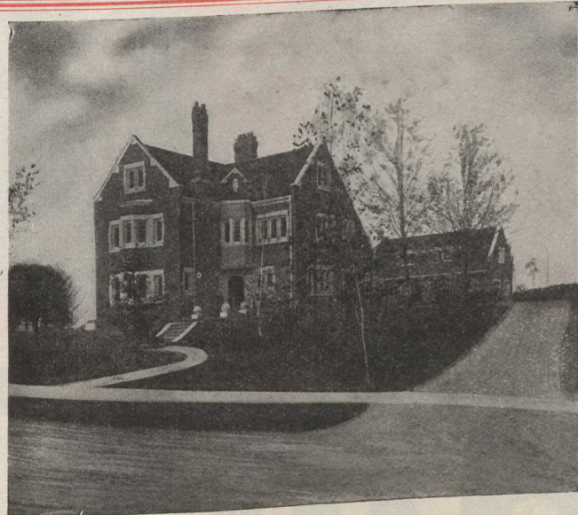
A Residence of Quality in Lawrence Park
