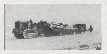
JT TRACTOR HAULING LOAD OF 24 TONS AT 20° BELOW ZERO.
