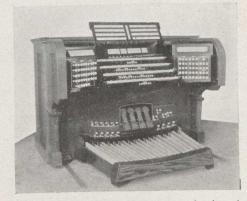
The "console" of a modern organ showing the four manuals, pedal keyboard, stops, combination buttons. balanced swell pedals, etc.
