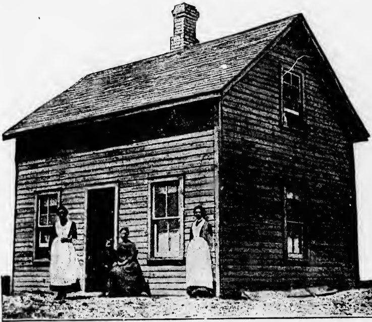
No. 5.—Cost $300 (£60).—This house, 20 x 16 ft., is divided into two rooms downstairs, and can also be divided into two rooms upstairs; cellar underneath, with trap door in kitchen floor.
