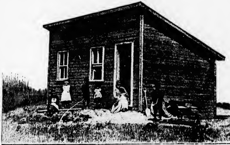
No. 4.—Cost $120 (£24).—This house has one room, 18 × 12 ft., cellar underneath, with trap door in floor.
