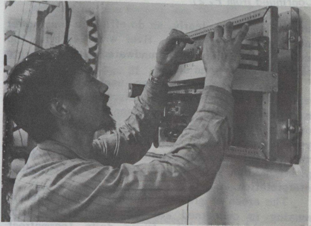
Willie Adams, a resident of Rankin Inlet, adjusts the Comminterphone conference unit in the telephone exchange building of a small northern community.
