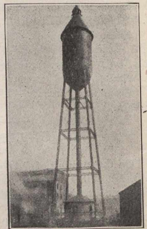
112,000 Gals.—162 ft. High. Lackawana Steel Co. Buffalo, N.Y.
