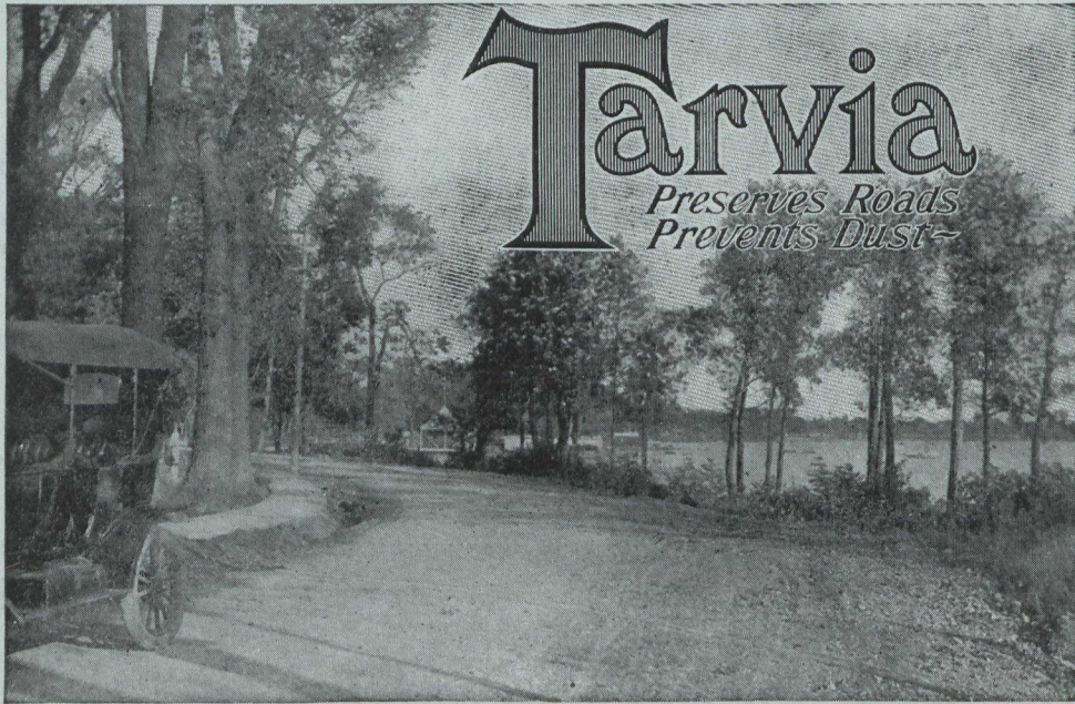
Pointe Claire Road, Quebec. Tarvia Filled Macadam.
