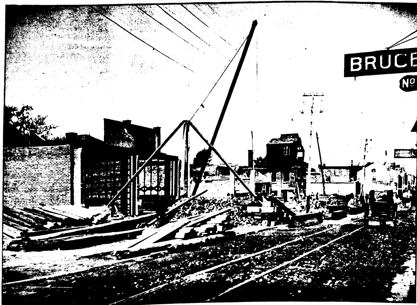
MONTREAL IMPROVEMENTS—WIDENING ST. LAWRENCE MAIN STREET. TEARING DOWN AND REBUILDING THE WEST SIDE.
