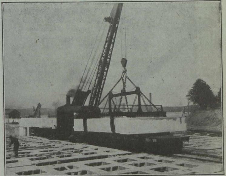
Crane Loading Block onto Flat Car. Note Specially Designed Lifting Tongs.
