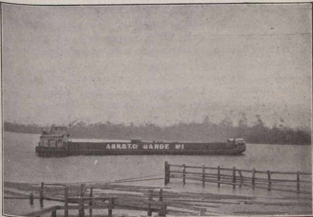
Fig. 1.—First of Fleet of Fifteen Barges, Propelled by Producer Gas Engines.
