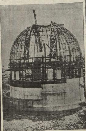
This slotted dome is t o shelter the telescope.
