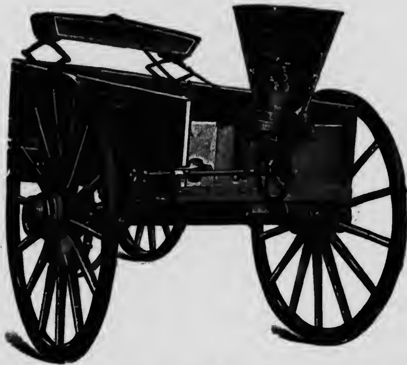
Fig. 2 Endgate Rotating Distributor, attached to rear of common Farm Wagon.
