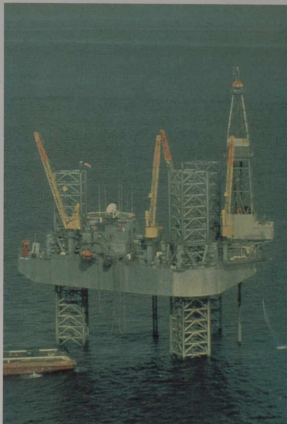
Drilling rig Rowan Juneau in the Venture field.
