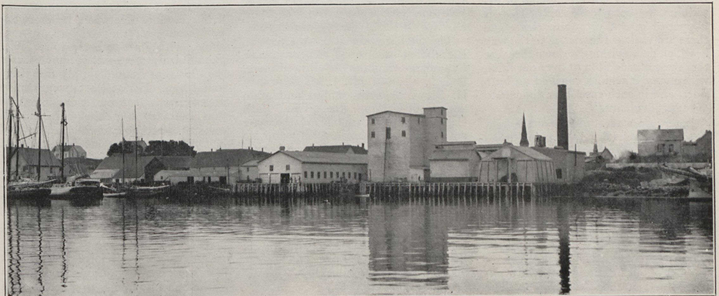
Fish Packing and Storage.—Plant of the Lockeport Company, Lockeport, N.S.
