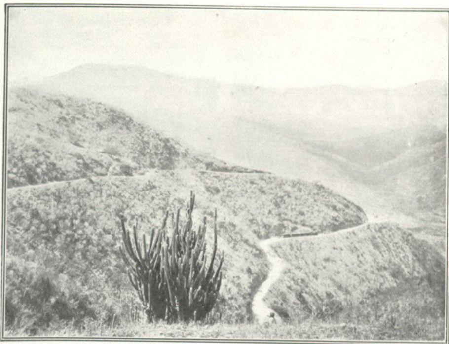
A VIEW OF THE FAMOUS LA GUAYRA AND CARACAS RAILWAY—A TRAIN MAY BE SEEN WINDING ITS WAY ALONG THE LOWER LEDGE
