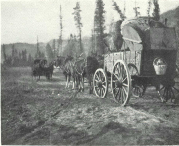
SUPPLIES ENTERING CANADA AT MIDWAY FOR THE V.V. AND E. CONSTRUCTION
