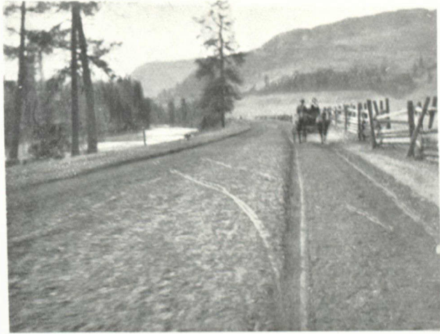
THE VALLEY OF THE KETTLE RIVER, WHERE THE V.V. AND E. WILL RUN. NEAR MIDWAY, B.C.
