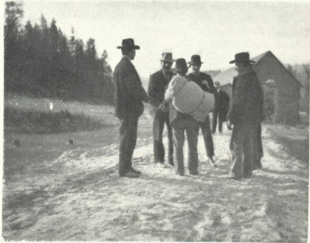
NAVVIES ENTERING CANADA AT MIDWAY TO WORK ON THE CONSTRUCTION OF THE V.V. AND E
