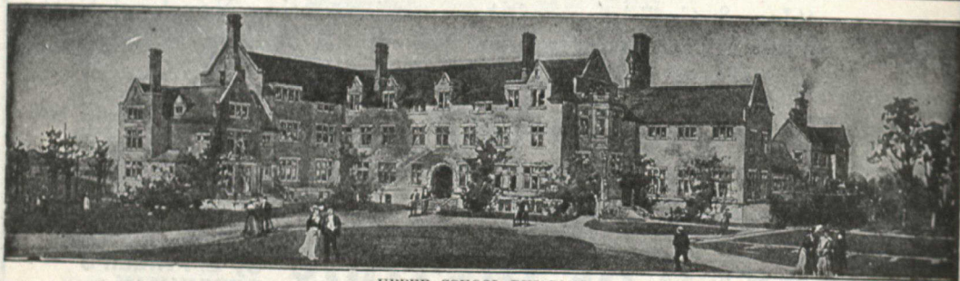
UPPER SCHOOL BUILDING
