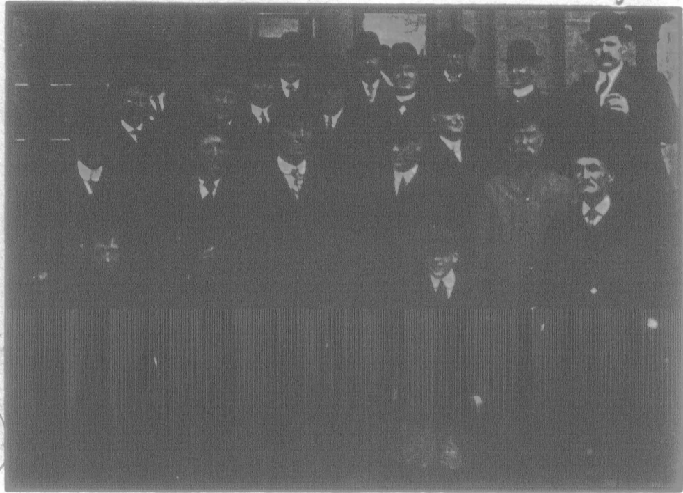
The Men Who Make Tile and Brick in Western Ontario.
