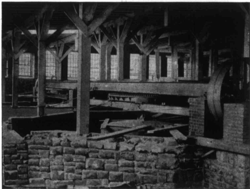
Marlbank Plant Two of the Wash Pits in course of construction
