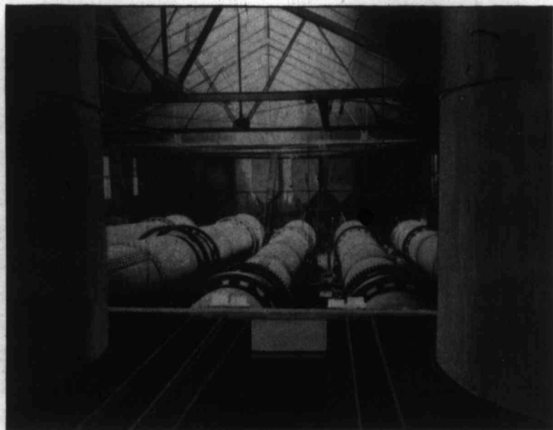
Marlbank Plant. Partial view of the Rotary Kilns
