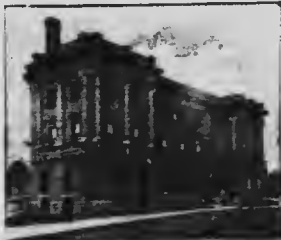
FRONT VIEW CITY DAIRY BUILDING SPADINA CRESCENT
