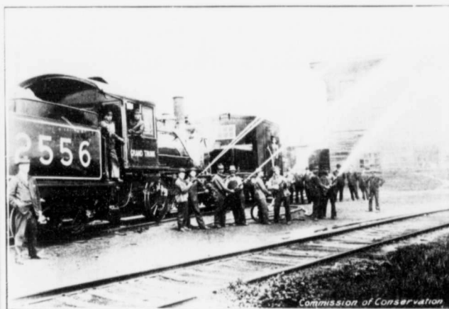
THE ABOVE TANK CAR BEING TESTED
