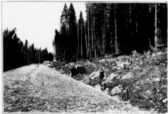
KETTLE VALLEY RAILWAY RIGHT-OF-WAY After piling and burning of debris. Vernon District, B. C.
