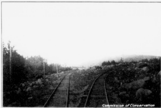
HEAVY FOREST GROWTH IMMEDIATELY ADJACENT TO NEWLY-CONSTRUCTED RAILWAY Note logs and small debris, from right-of-way clearing, piled at edge of timber. A small grass fire on the right-of-way might, by igniting this material, cause great damage to green timber before men could reach the scene and control the fire. Ontario.
