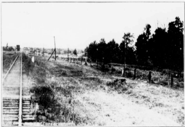
RAILWAY RIGHT-OF-WAY AFTER THE CUTTING OF GRASS In accordance with section 297 of the Railway Act. Fire danger greatly reduced. Ontario.
