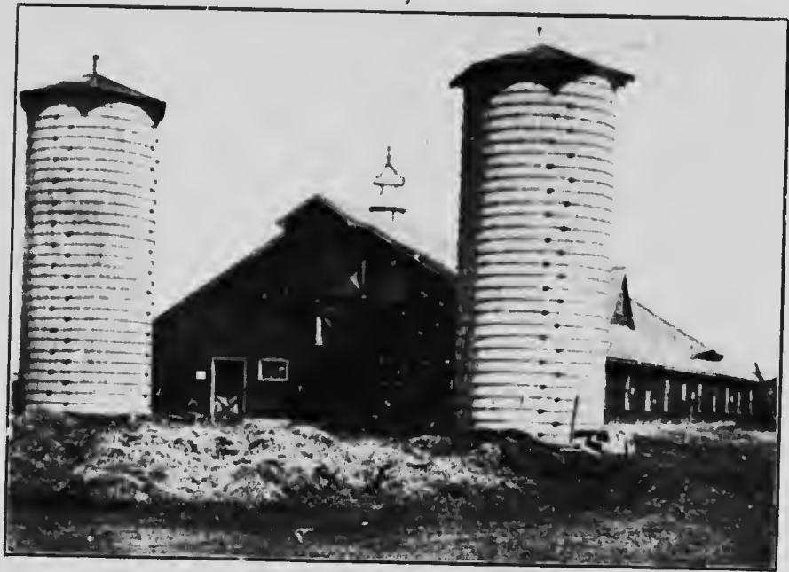
Cement Stave Silos, on Glenlea Stock Farm
