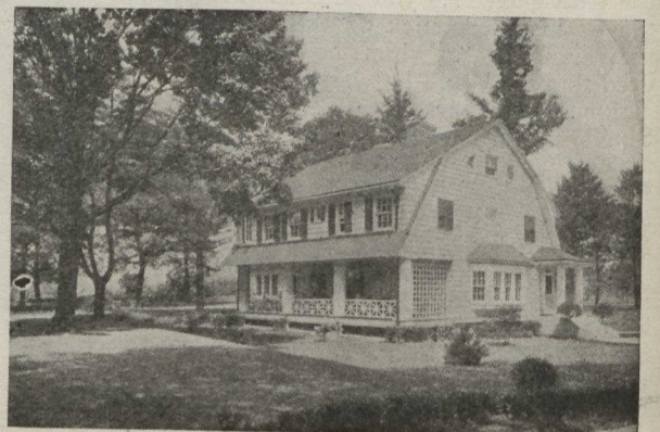
In this house the second floor is made larger than the first by carrying the roof and long dormer out over the side porch.
