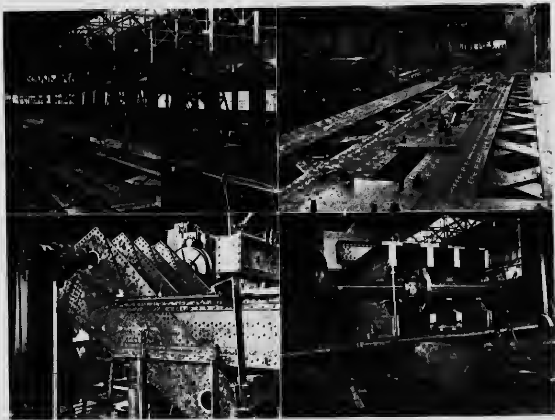
10 Views showing the interior of the shops with bridge members in the process of manufacture
