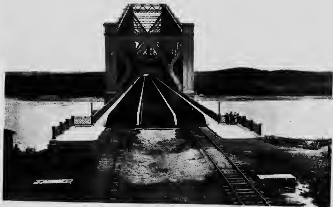
78 End view of the Bridge
