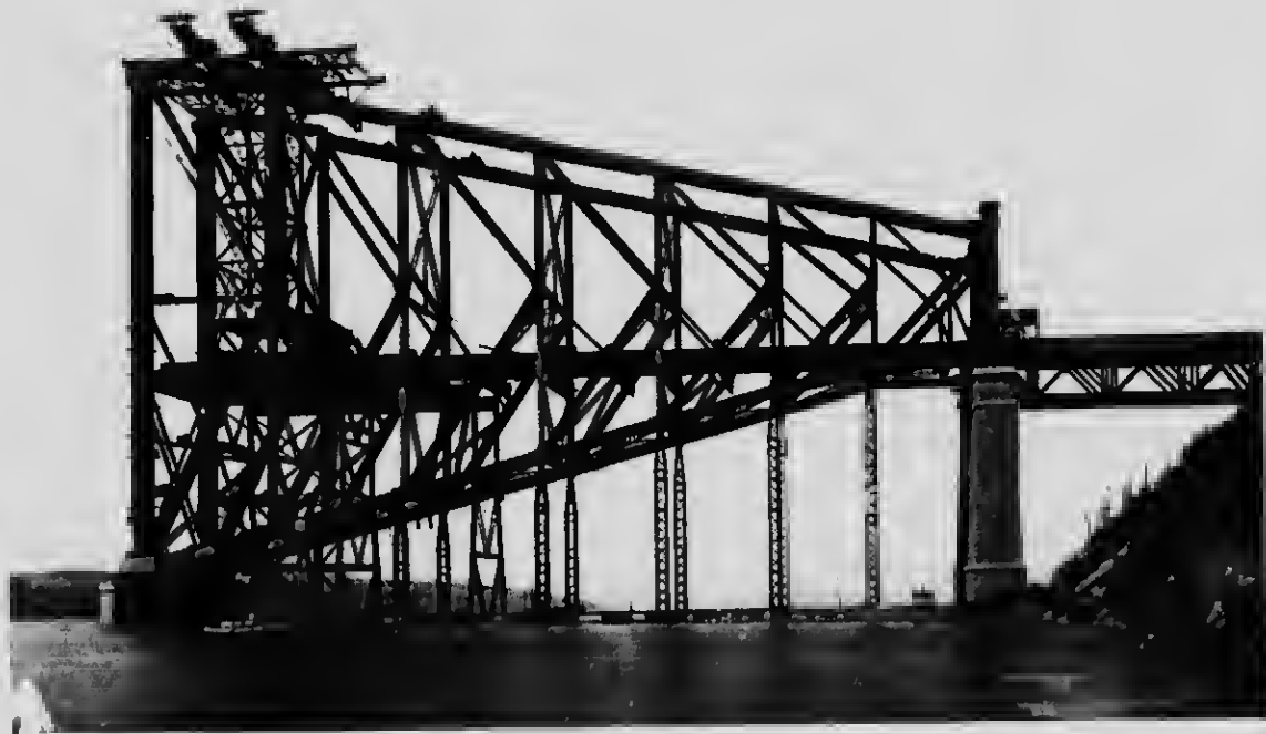
30 The erection of the North Shore anchor arm completed June 7th, 1915
