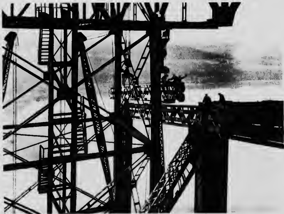
39 Placing the upper chord members of the cantilever arm
