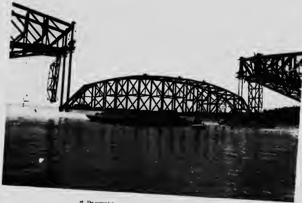
66 The suspended span carried by the hoisting chains; scows floating out
