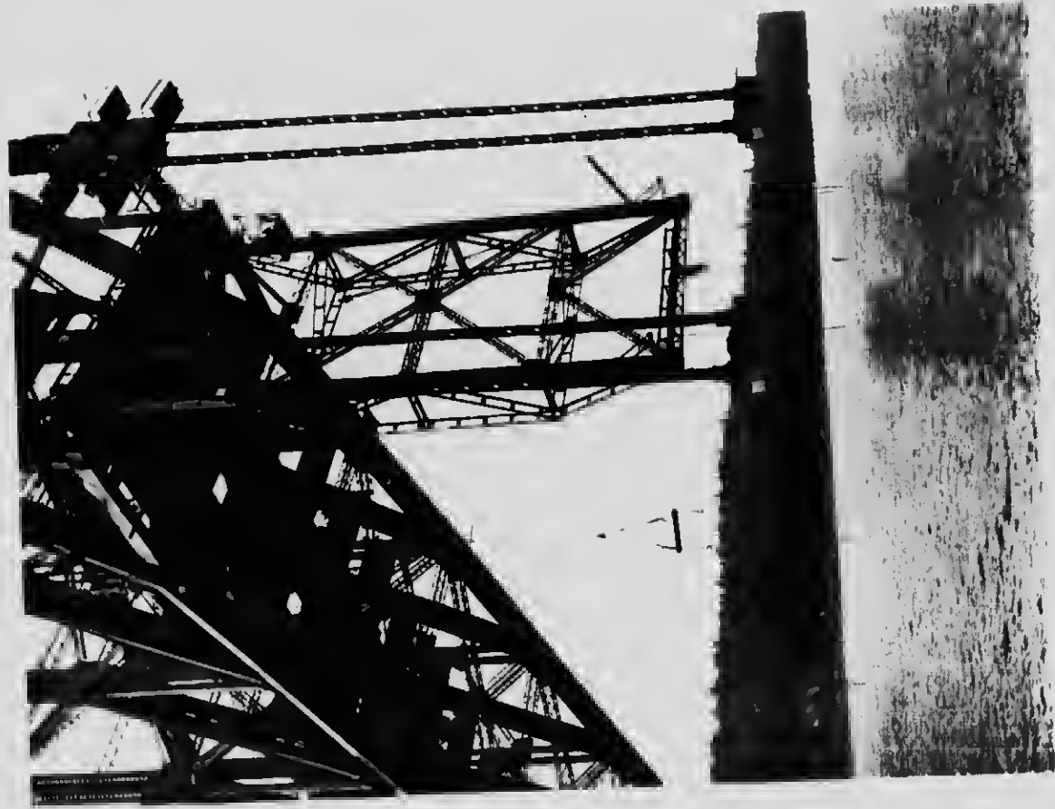
63 The chains and mounting frame after the loss of the suspended span
