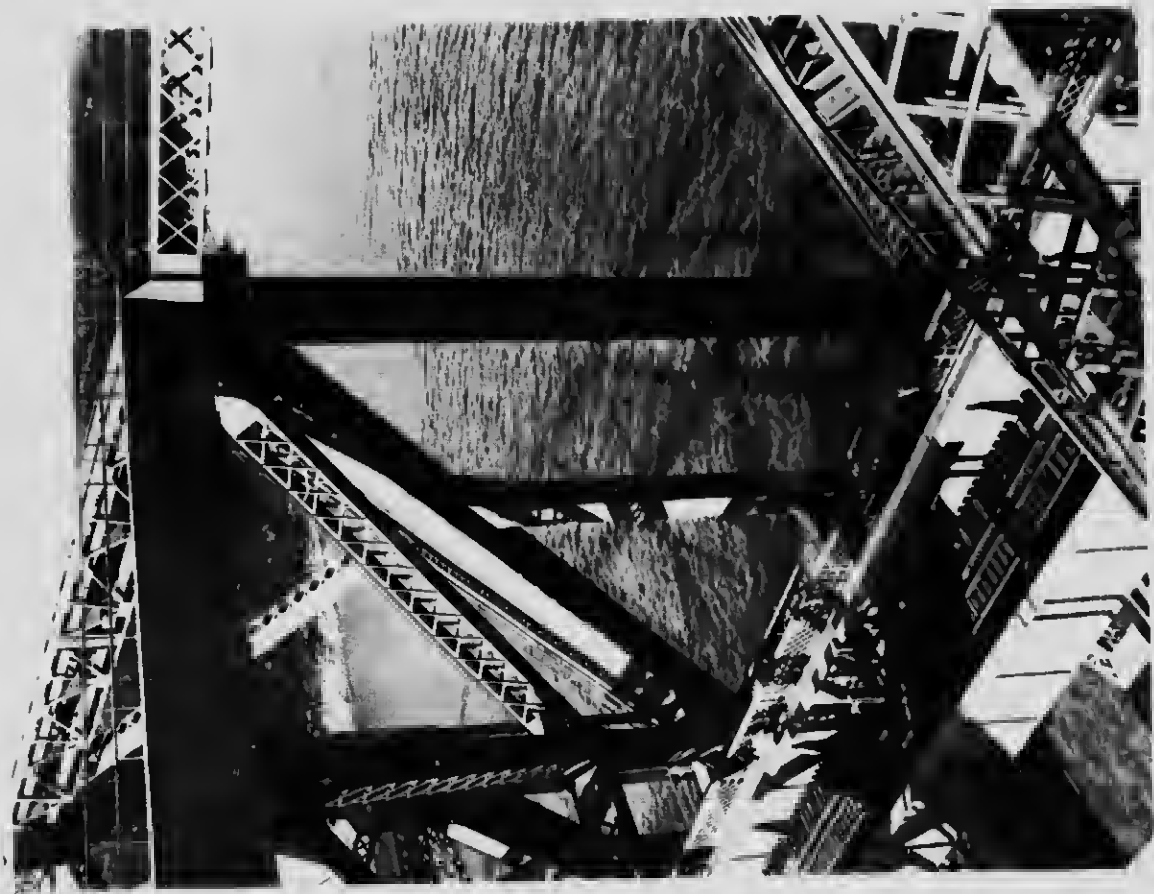
71 Pychar Hanger supporting one corner of the suspended span from the end of the cantilever arm
