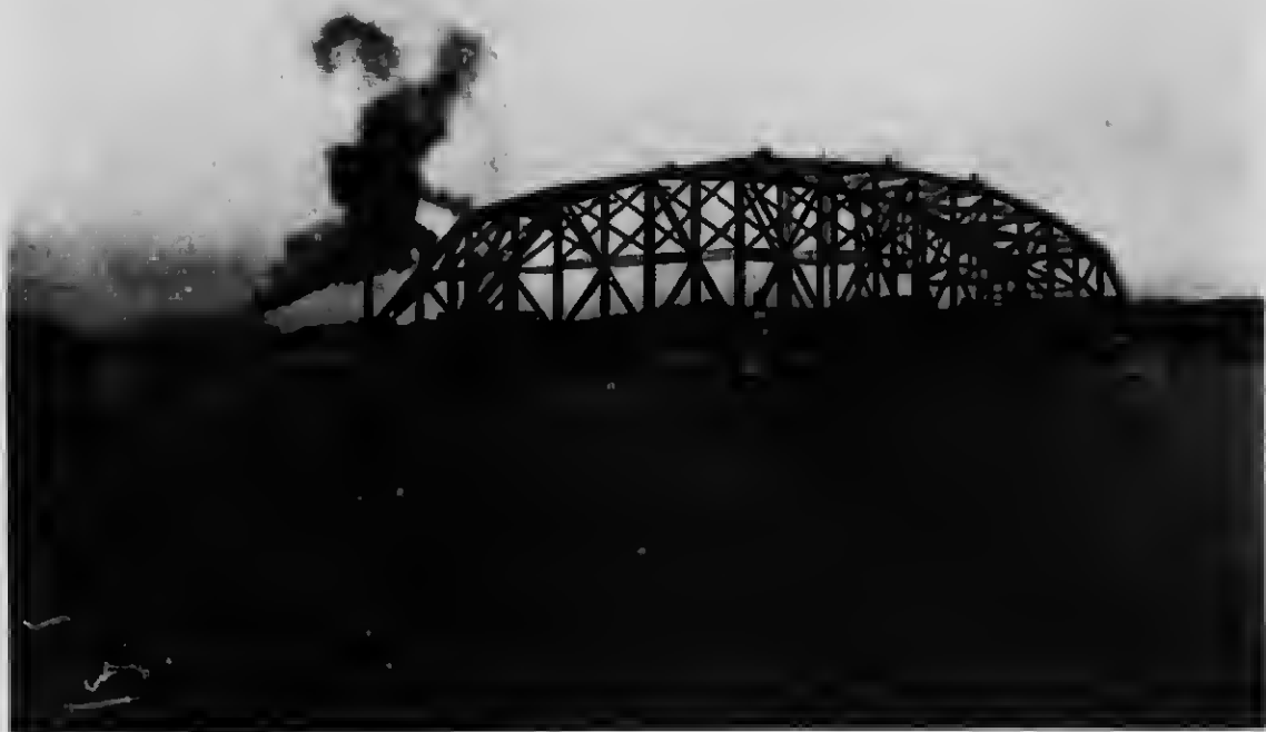
57—The suspended span being guided up the river
