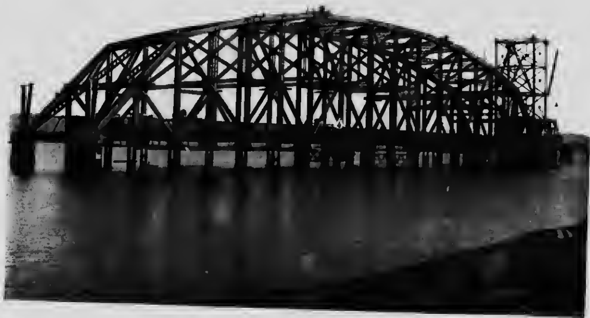
46—The suspended span erected on falsework at Sillery
