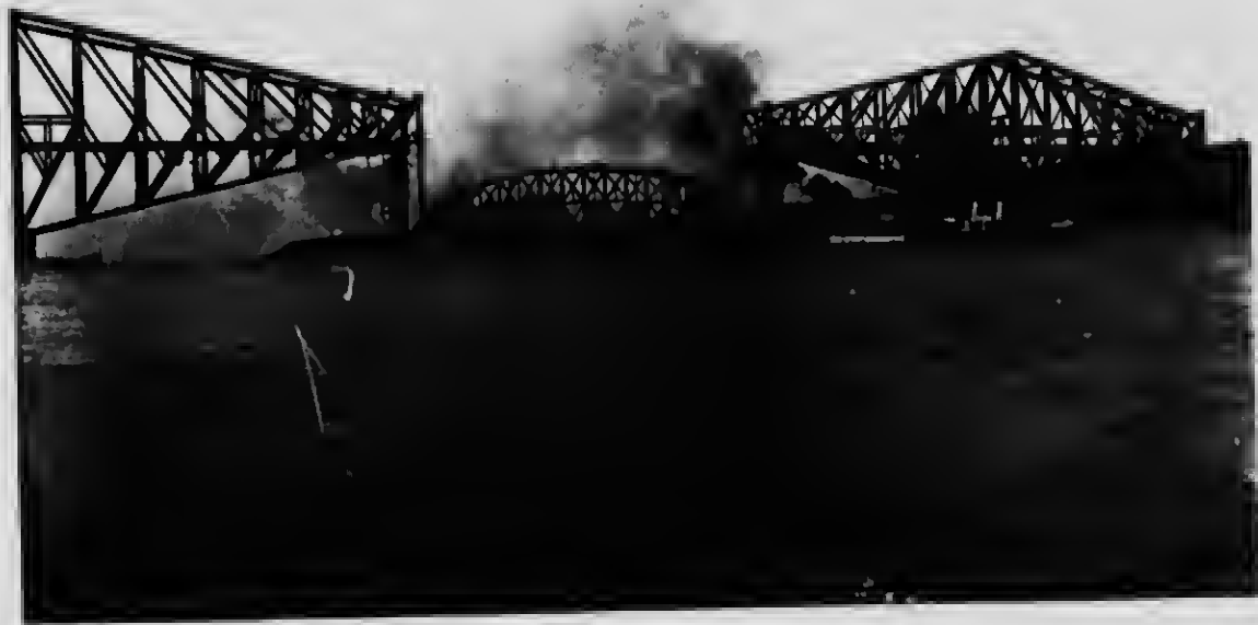
61 - September 11, 1916. 10 40 a.m. Just before the loss of the suspended span
