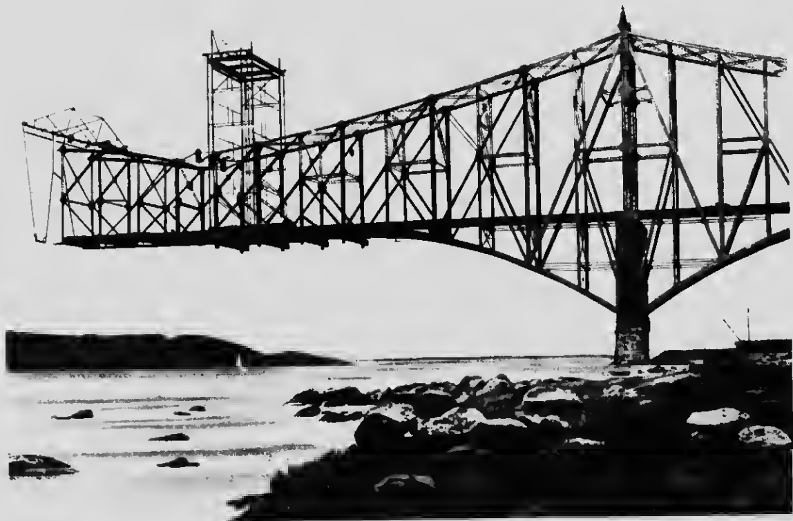
4 Photograph of the Phoenix Company's bridge taken August 28, 1907, showing condition of the structure just previous to its failure
