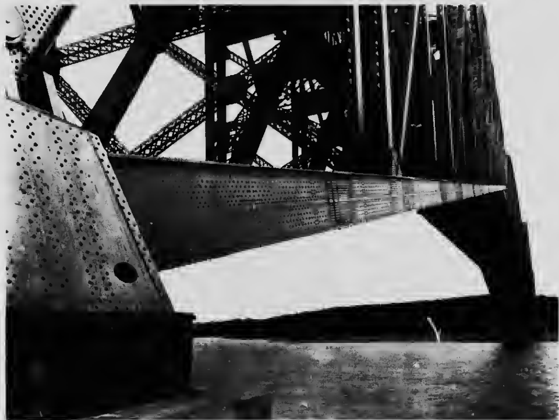
77 View of the Channel Span from one of the Main Piers
