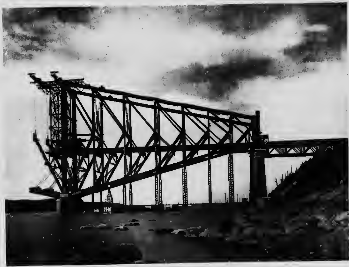
32 Half panel of the cantilever arm erected with the members of the outer half of the panel in place
