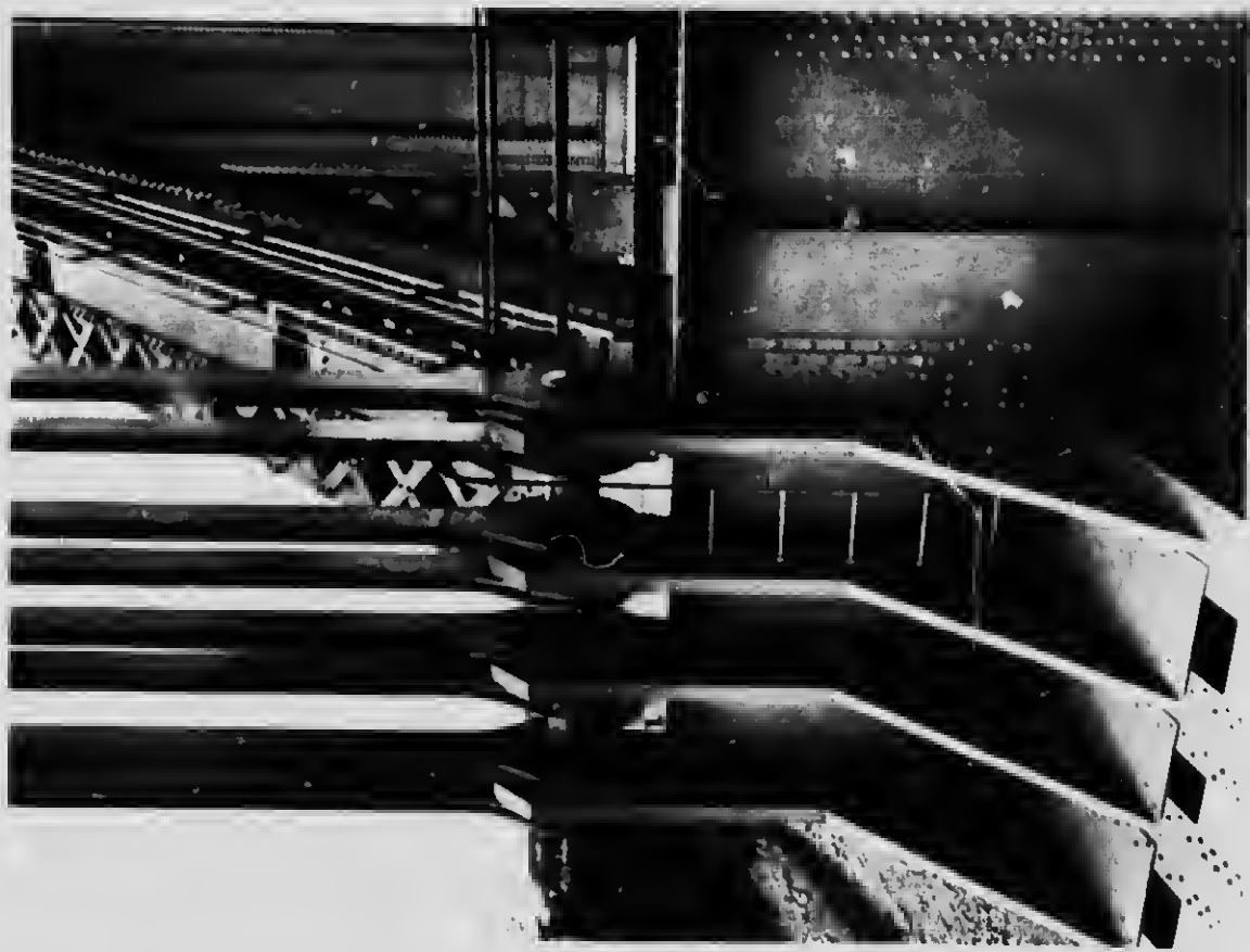
75 - Detail at A.L.2. showing the floorbeam connection to the outer end of the Anchor Arm bottom chord
