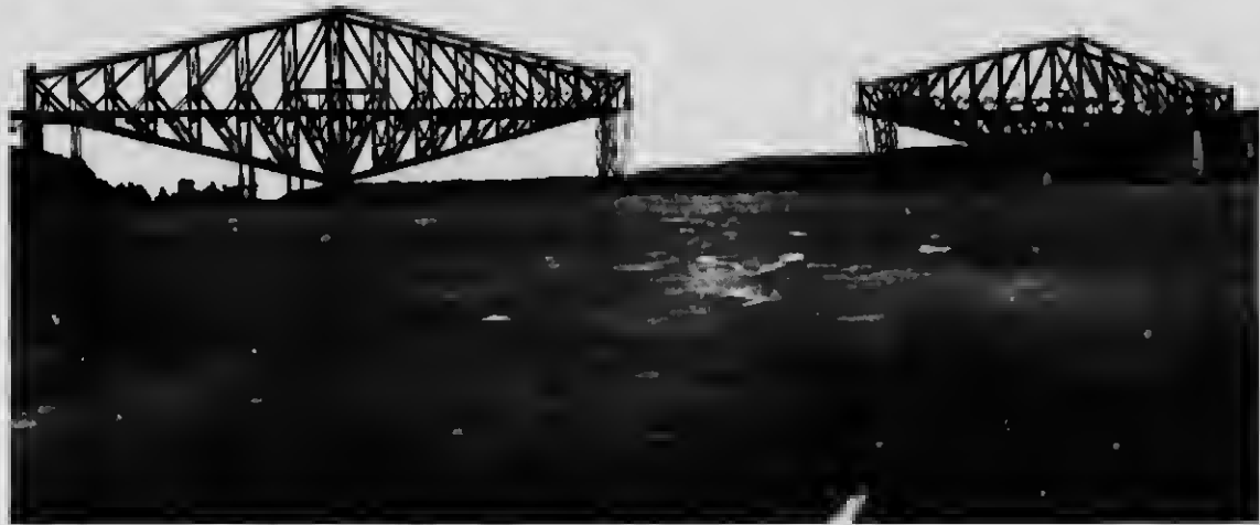
47 - Progress of erection, August 11, 1916
