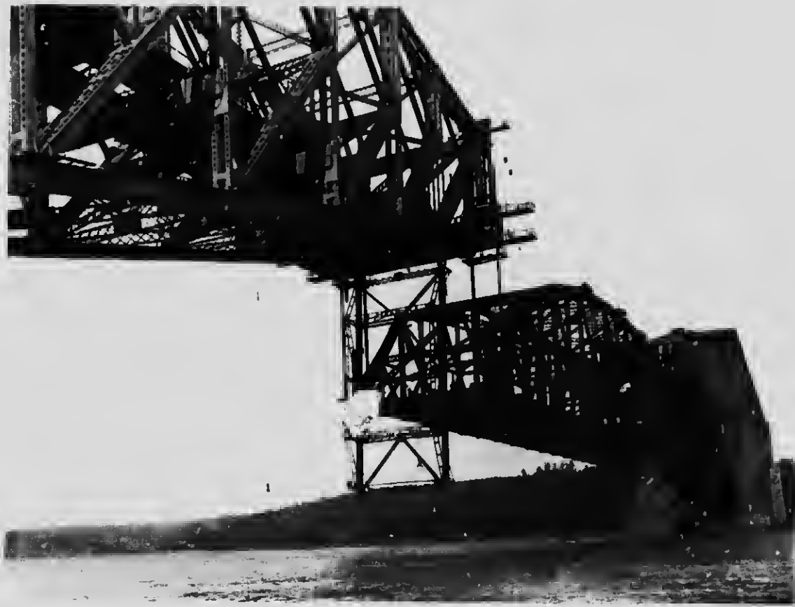
66 The suspended span about half way up, September 18th, 1917
