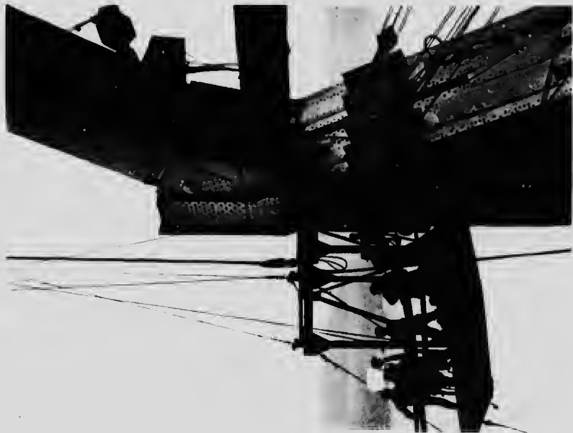
31-Connecting the first panel of the castliver crane
