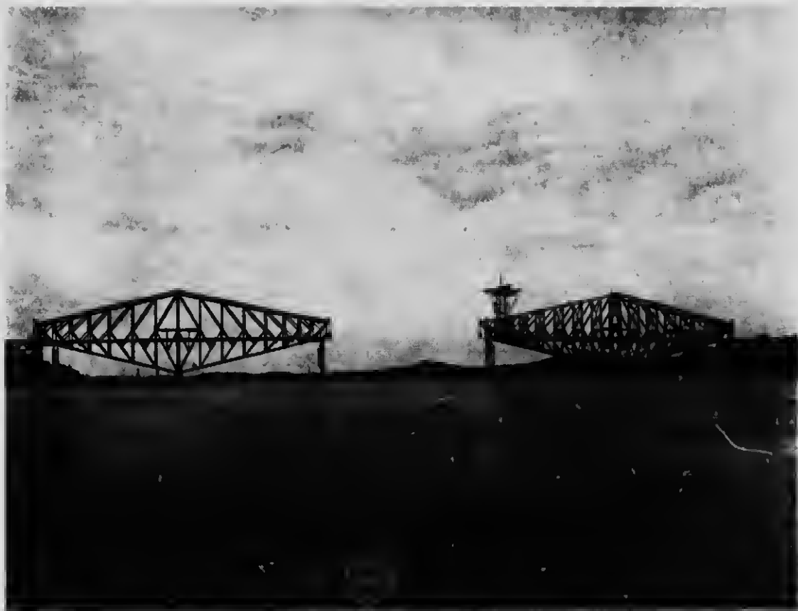
46—Cantilevers completed, hoisting apparatus partly assembled
