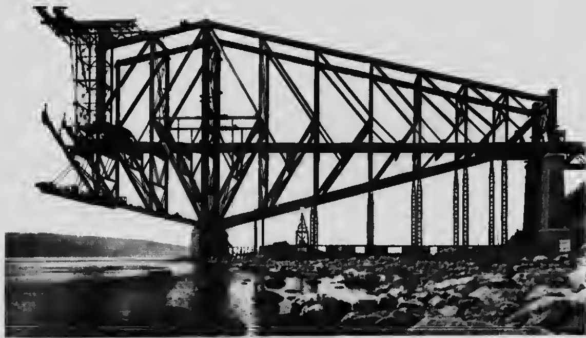
36 Erecting the third panel of the cantilever arm
