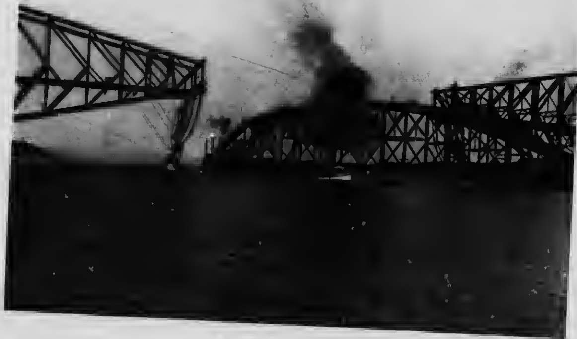
58—The suspended span being guided to position
