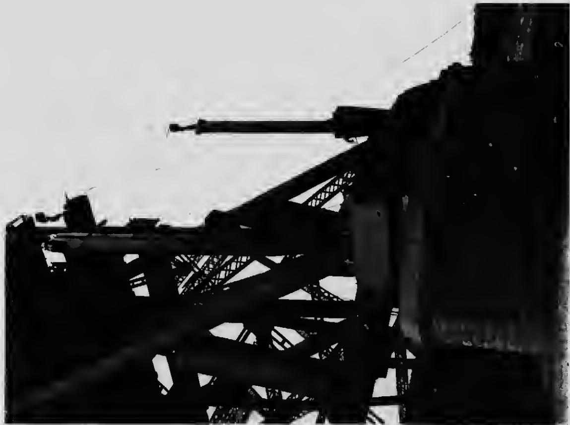
23. Starting the erection of the anchor arm web system
