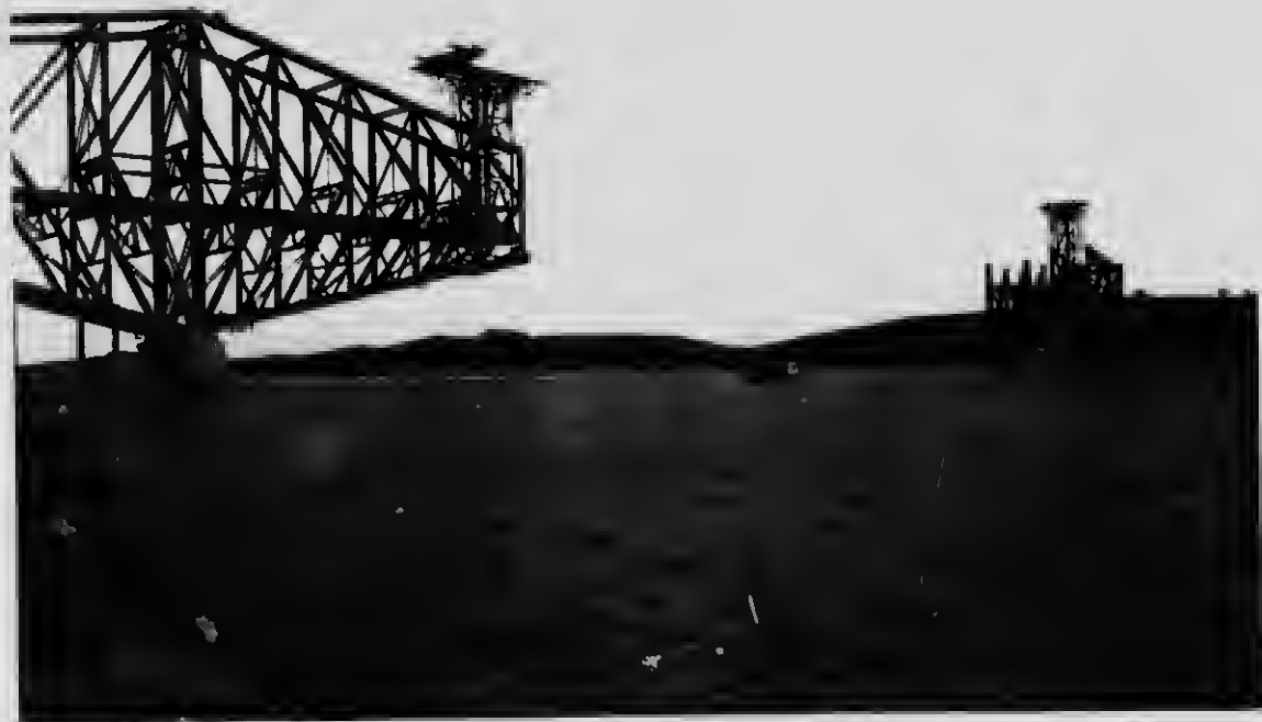
43 Progress of erection, September 10, 1915
