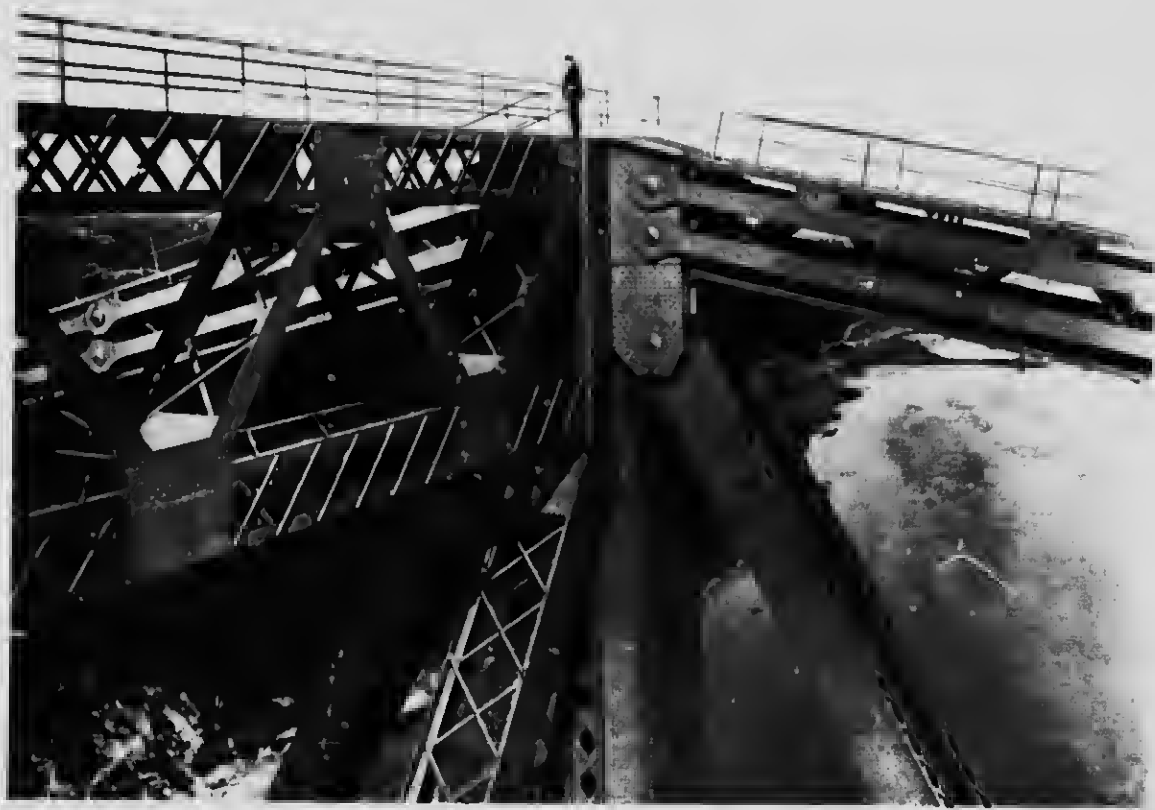
72 Detail at the top of the Main Post
