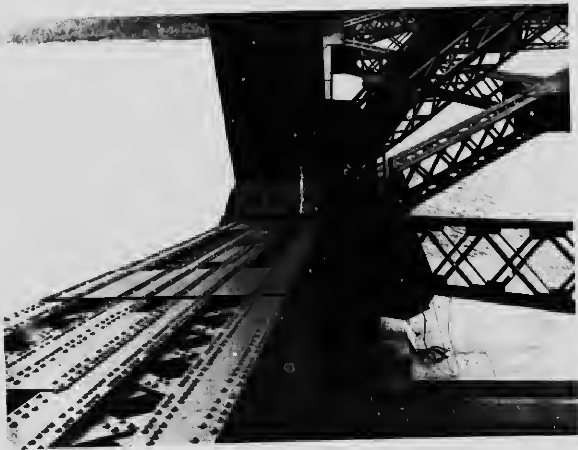
73 View showing the connections to one of the Main Pier shoes
