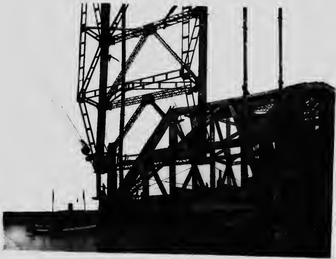
59 - The suspended span moored. Note the mooring ropes, also the hoisting chains being connected.
