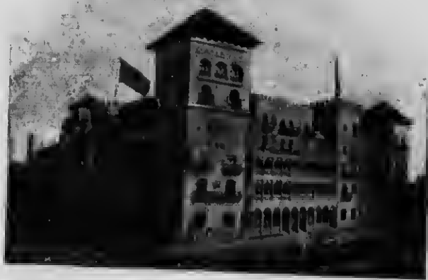
The Casa Monica is the finest monolithic cement hotel in the world, and a substantial demonstration of the durability, beauty and cheapness of concrete construction. Face frontage, 400 feet; tower, 100 feet high; balconies, arches, cornices, battlements, walls, floors, ceilings, all of Portland Cement concrete. This hotel was built in 1887.
