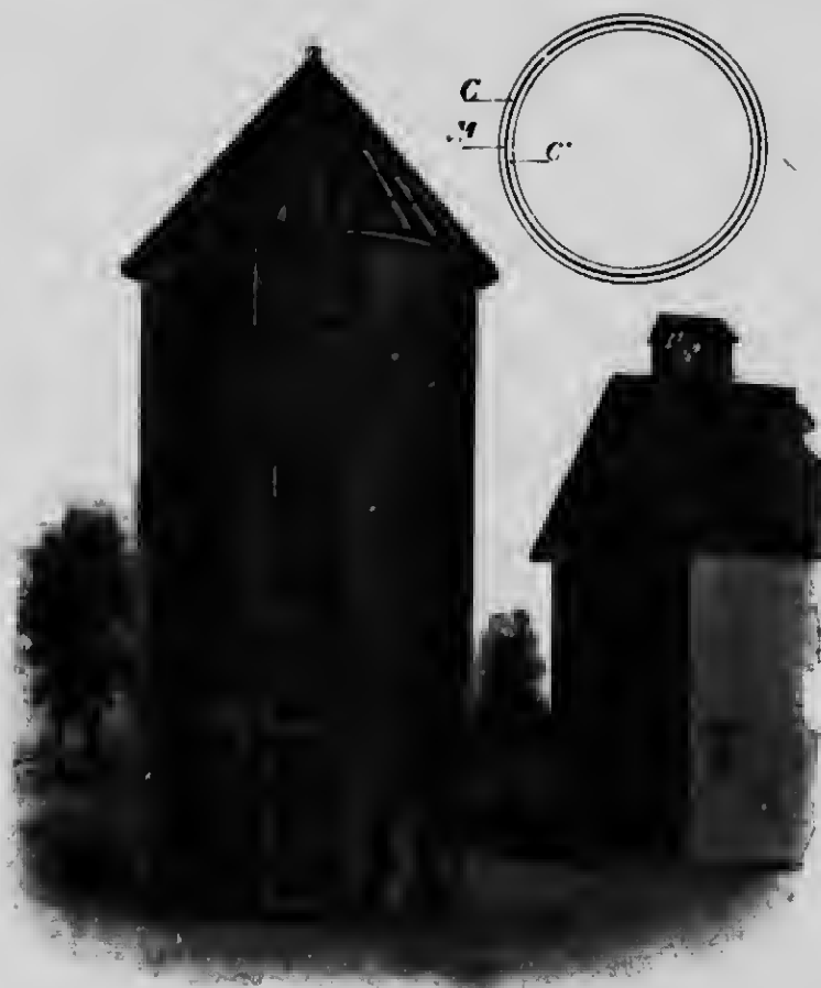
A PORTLAND CEMENT SILO.
