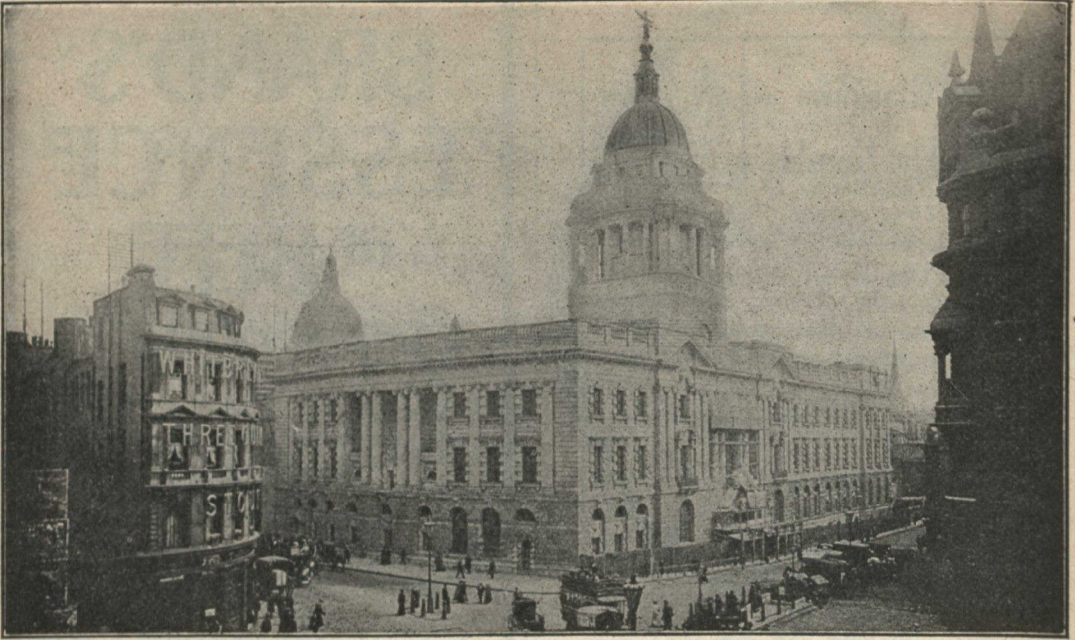
The new Bailey is worthy of the greatness of modern London and takes rank with the great palaces of justice for which Europe is celebrated. Frontage, 237 ft. (Old Bailey) and 142 ft. (Newgate St.); average height from pavement to top of balustrade, 75 ft.; height of dome to the ball, 195 ft.; bronze figure of Justice, 12 ft. high; civic sword held by statue, 6 ft. long. Figures over entrance representing "The Recording Angel," "Truth" and "Fortitude," sculptured by Mr. F. W. Pomeroy, A.R.A.
