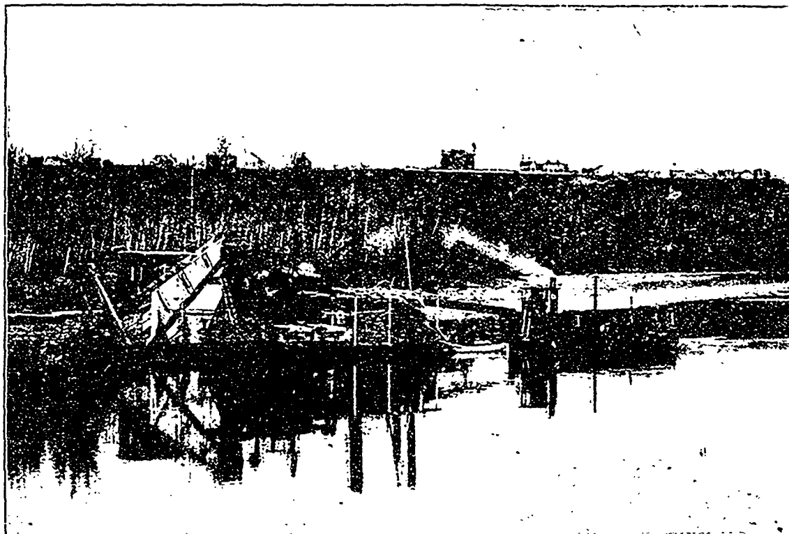
Showing the type of Dredge working on the River.
