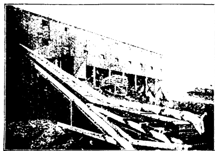
Freight and Package Elevator
