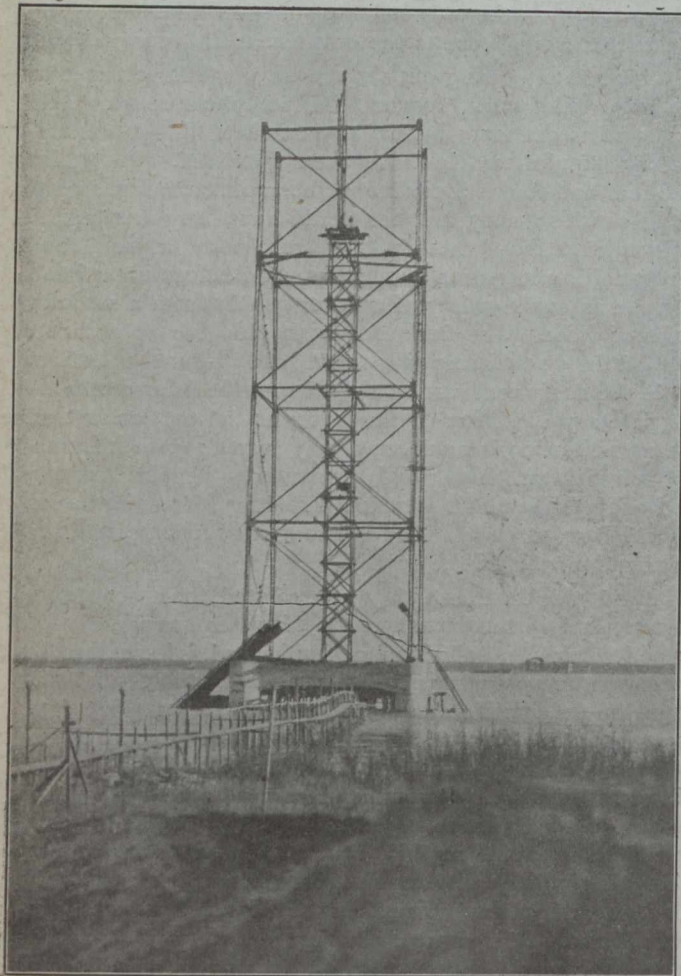
Fig. 1.—Steel Tower on North Side of St. Lawrence River
