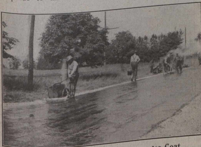
Fig. No. 5.—Putting on the Squeegee Coat
