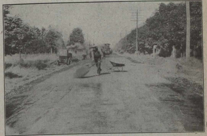
Fig. No. 6.—Sanding Over the Squeegee Coat
