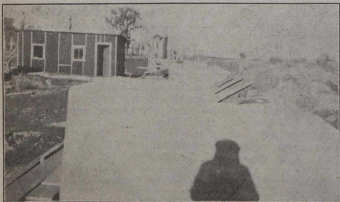
Fig. 2.—Anchor Piers, Behind Steel Towers
