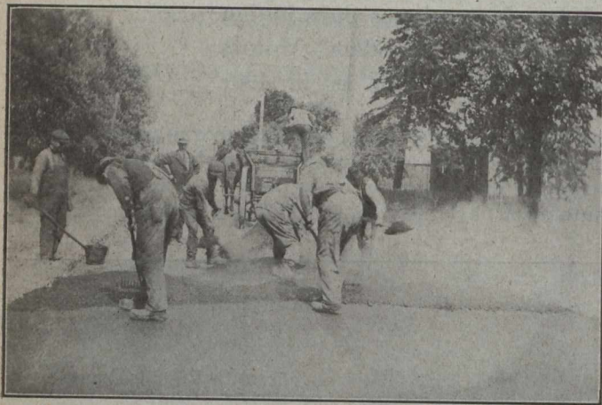
Fig. No. 3.—Raking the Hot-mixed Material with Hot Rakes. Material in Foreground Has Been Rolled
