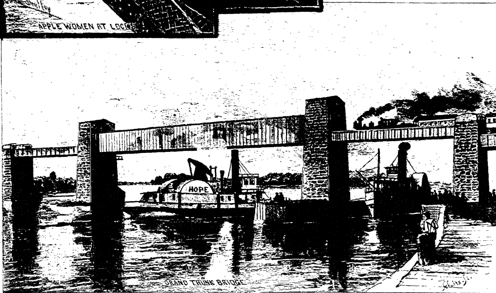
CANAL LOCK, AND RAILWAY BRIDGE AT STE. ANNE'S.
