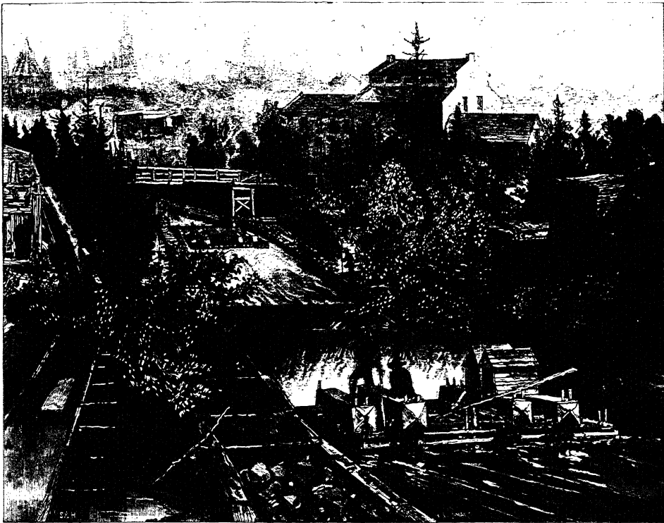
CRIB OF TIMBER RUNNING THE SLIDE.
