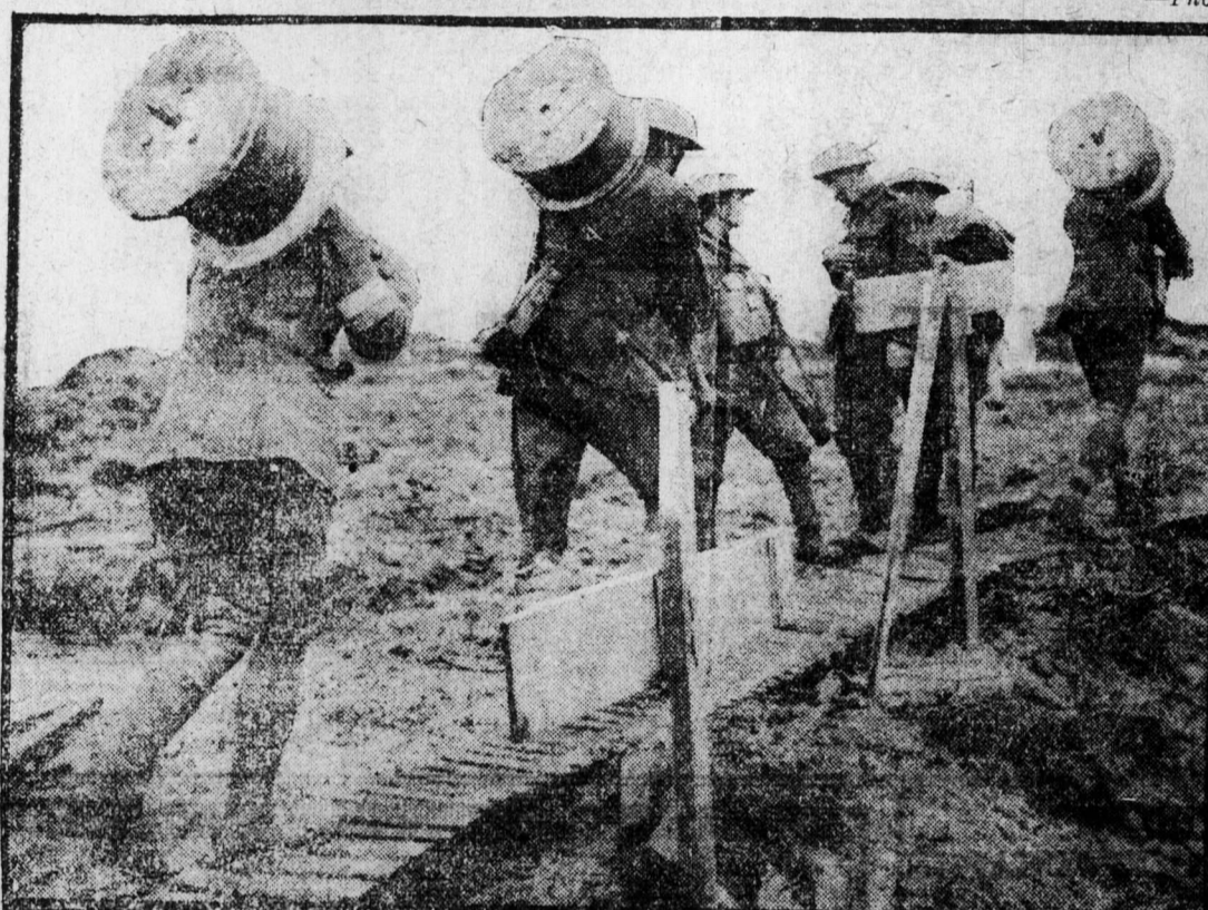
The Battle of the Ridges.—Telegraph wire going up for no man's land. Signallers on the way to establish communications.
