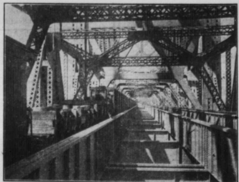
The Big Quebec Bridge, carrying 55 cars and two engines, weighing 7,000,000 pounds. Half a load for the Bridge.
