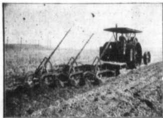
20-H.P. I H C Tractor Pulling 6-Bottom Plow
