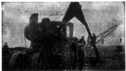
And besides plowing, house moving and road grading, here is another kind of work you can do. We build a shovel attachment for the Avery Undermounted Engine as shown here. With it you can dig drainage or irrigation ditches, load gravel, strip coal and do other work. You can get more attachments with an Avery Undermounted Engine for doing more different kinds of work than with any other engine.
