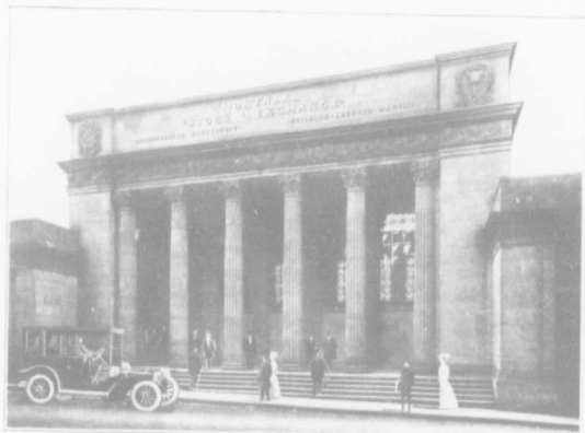
MONTREAL STOCK EXCHANGE BUILDING
