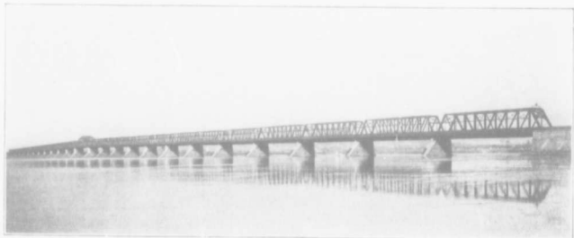
VICTORIA JUBILEE BRIDGE, MONTREAL
