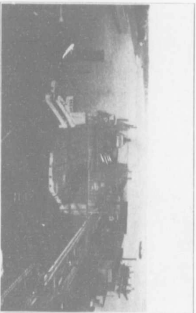
Grain Elevator No. 2. First entire concrete elevator in the world. Capacity 2,622,000 bushels.
