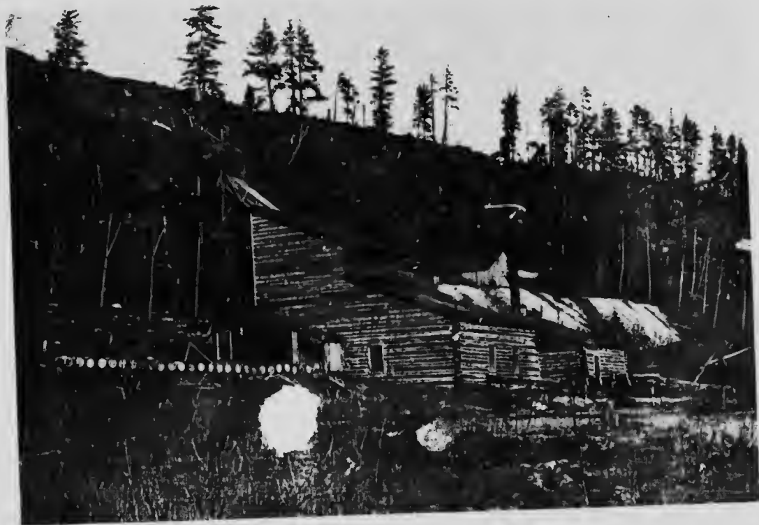
STAMP MILL AT WEST END MINE
