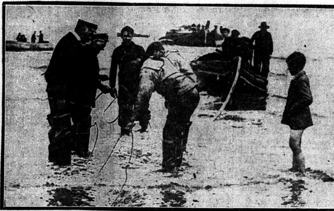
Bringing the world's largest ocean cable ashore at Weston, on the English coast. The other end is in New York.
