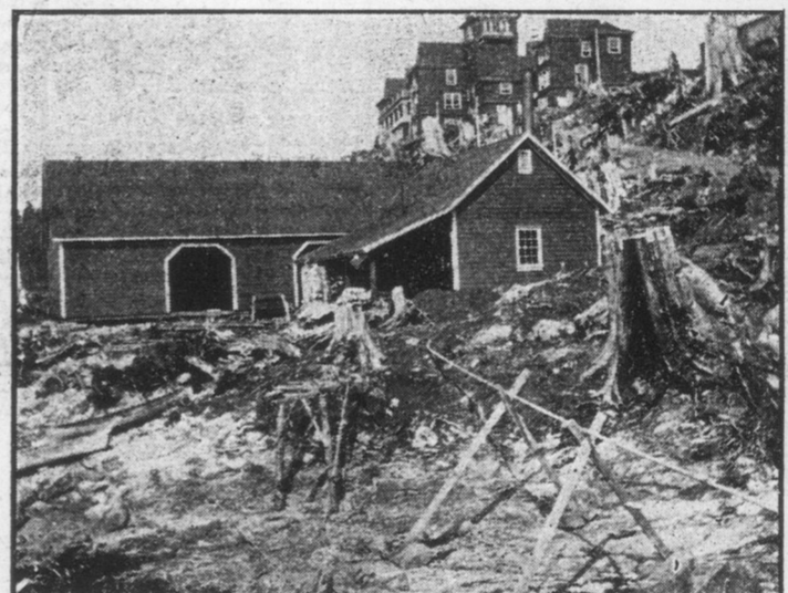
PUMPING STATION AT BAMFIELD CREEK.
