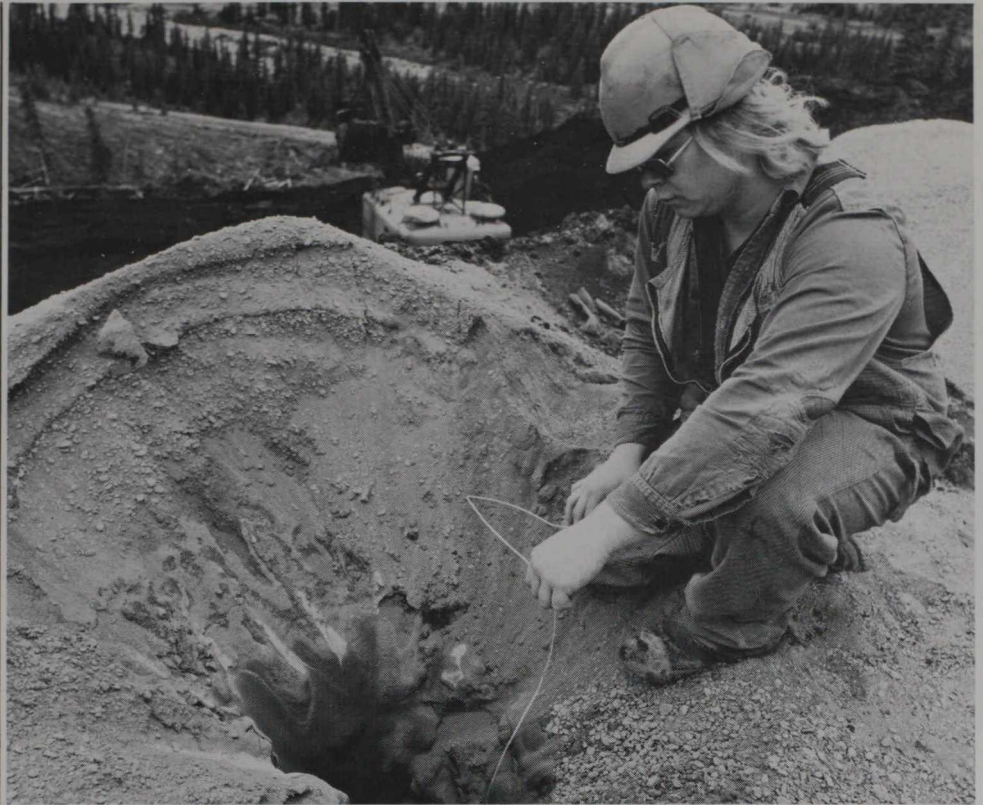
Surface mining at Hinton, Alberta: a mine worker measures the depth of a hole before filling with explosives.
