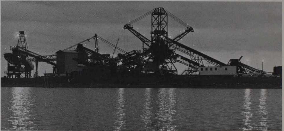
Complex coal loading equipment stands on reclaimed land at Roberts Bank Superport, British Columbia.
