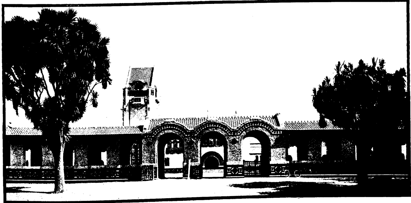
Detail of Entrance, State Normal School, San Jose, California. The largest concrete building of its kind in the world, and the most notable monolithic structure ever erected in America. The exterior of the rough walls are covered with a pebble dash of "Medusa" White Portland Cement. From an artistic standpoint nothing has thus far been developed in this particular type of structure to equal it. Because of its immense proportions and unusual treatment it is attracting world wide attention.
