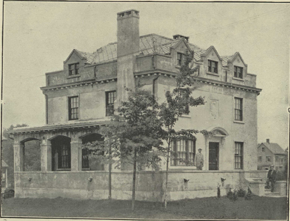
Solid Reinforced Concrete Residence erected by the American Building Corporation at Montclair, N.J.
