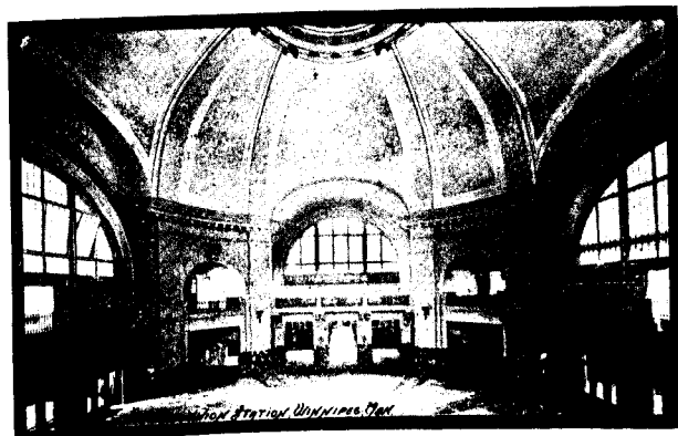
Rotunda, New Fort Garry Union Station, Winnipeg, Man.
