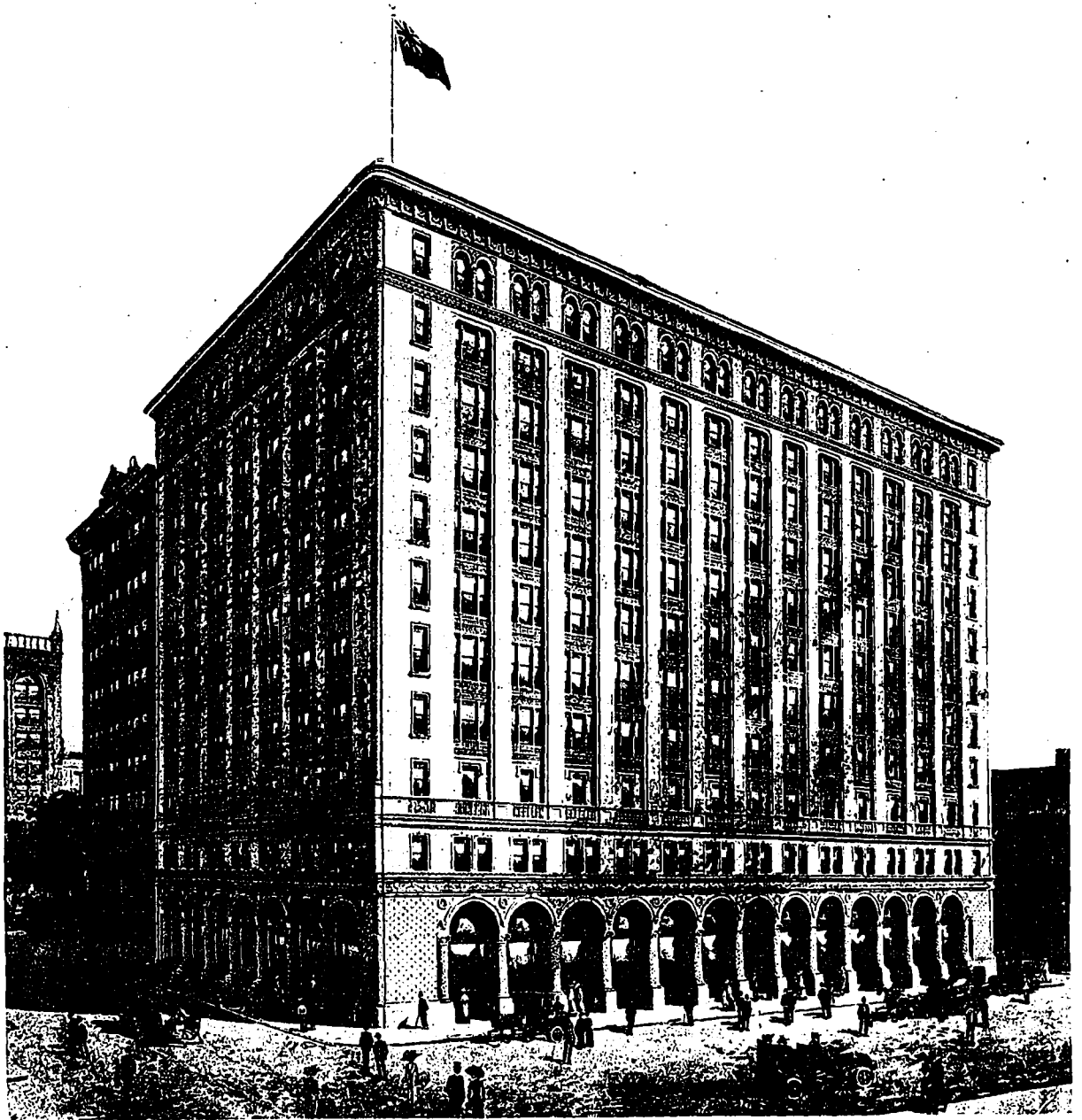
Perspective View of the Transportation Building now in Process of Erection at Montreal, and Which Will be a Notable Addition to the Many Imposing Buildings of the Business District. It will Occupy a Site Bounded by St. James, St. Francois Xavier, and Notre Dame Streets, Covering an Area of Approximately 20,000 Square Feet. The Building is to Be As Fireproof as Modern Science can Devise, with Steel Frame and Semi-glazed Terra Cotta Exterior. The Entire Ground Floor, Together with a Mezzanine, is to be Finished in Marble, and has Been so Arranged as to give Ideal Accommodations for Banking and Office Purposes. A Feature of the Plan is a Broad Arcade Extending Through the Ground Floor from St. James St. to Notre Dame Street, with an Intersecting Corridor Leading to the St. Francois Xavier Street Entrance, and Having a Monumental Staircase, Giving Easy Access to the Upper and Lower Floors. Carrere and Hastings and Ross and MacFarlane, Associate Architects.
