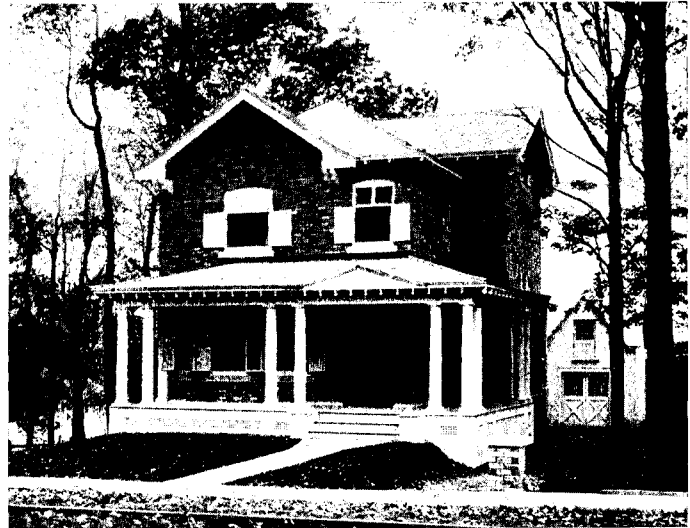
Residence of O. Normandin, Esq., Maplewood Avenue, Montreal, P.Q., Roofed with Asbestos Cement Shingles, No. 8 Gray (12"x12") with Red Ridge Roll.
