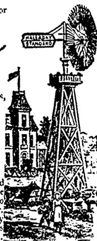
These celebrated Windmills are made from one man to forty horse-power. They are perfectly controllable in gales and uniform in speed. Geared Mills for chaff-cutting, root-pulping, threshing, sawing wood, grinding corn, etc., etc.
