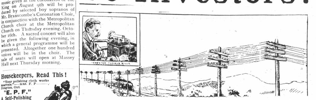
The Electrograph is a simple, practical machine for sending pictures, newspaper illustrations, maps, etc., by telegraph over the wires of sany telegraph or telephone company.
