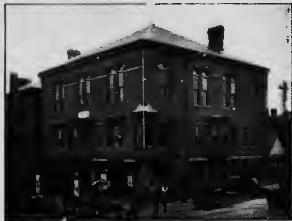
BOSTON MARINE BUILDING, YARMOUTH, N. S.
