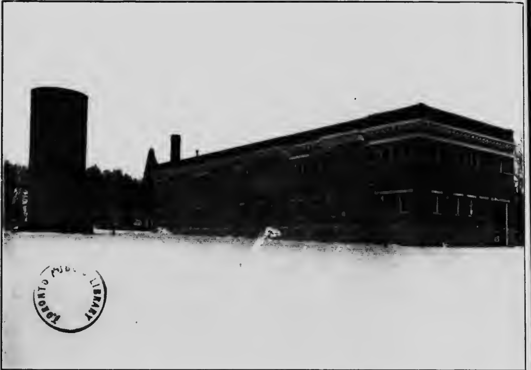
Niagara power in Toronto—The Transforming Station.
