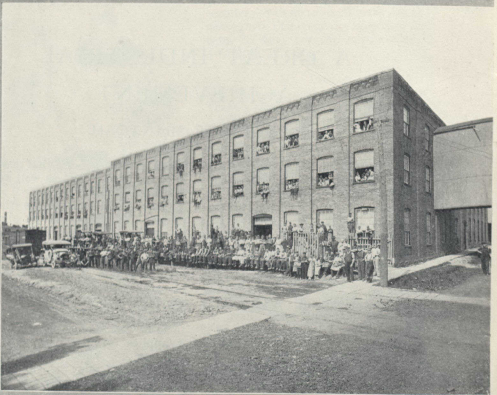
A PANORAMIC VIEW OF THE The camera stood in front of the general offices, and was pointed first to the right and then to the left.
