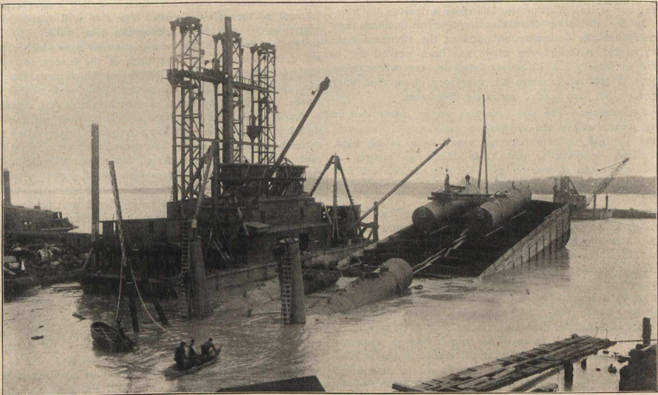
Lowering the First Section for the Detroit River Tunnel.
