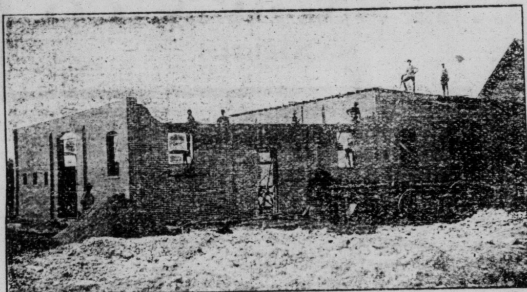
Power House in Course of Construction
