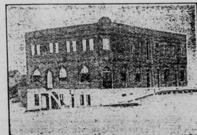
The Cahoon Hotel and Union Bank of Canada
