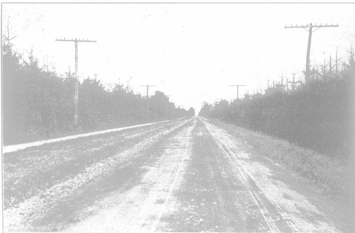
A Well-graded Road Which is Good in Fall and Spring.
